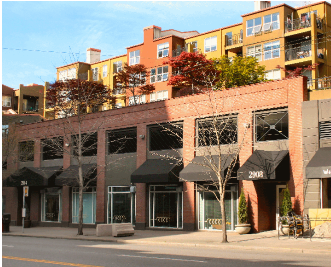
Figure 18.120.040.I.2.b. This building uses openings on its second level parking area to resemble windows.
