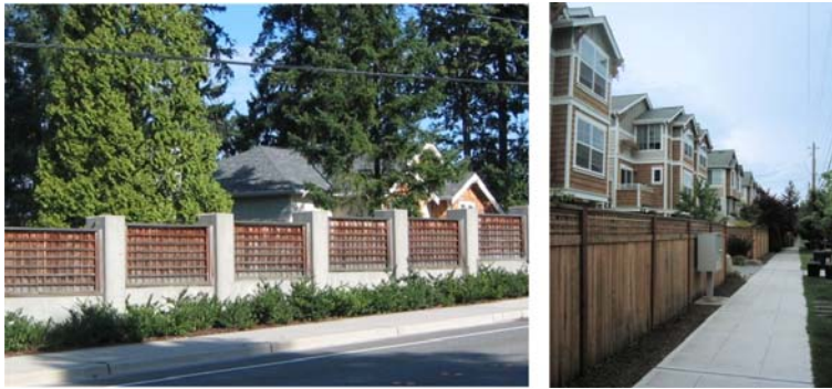
Figure 18.120.020.H.2.b. Fences that prevent visibility from public ROW and open spaces can decrease security.
