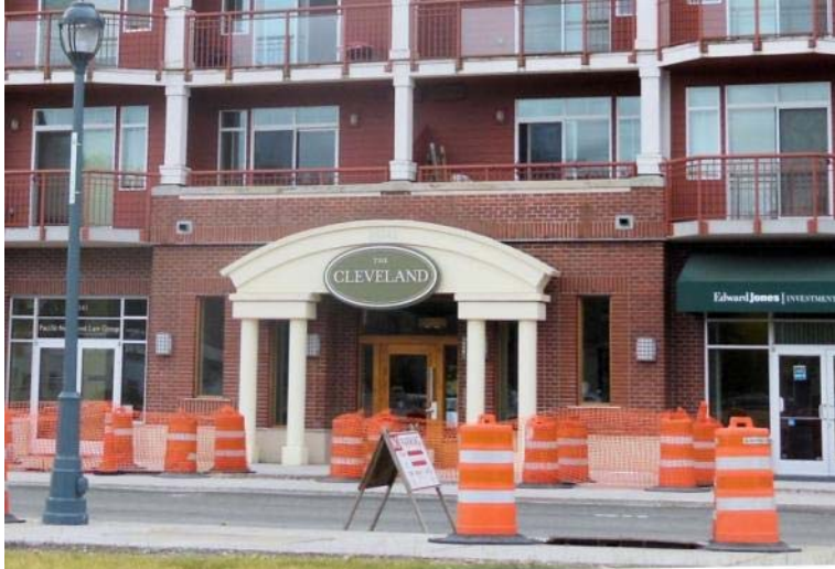
Figure 18.120.040.E.2.f While emphasizing the entry is laudable, the classical arch and columns clash with the other more contemporary façade elements.
