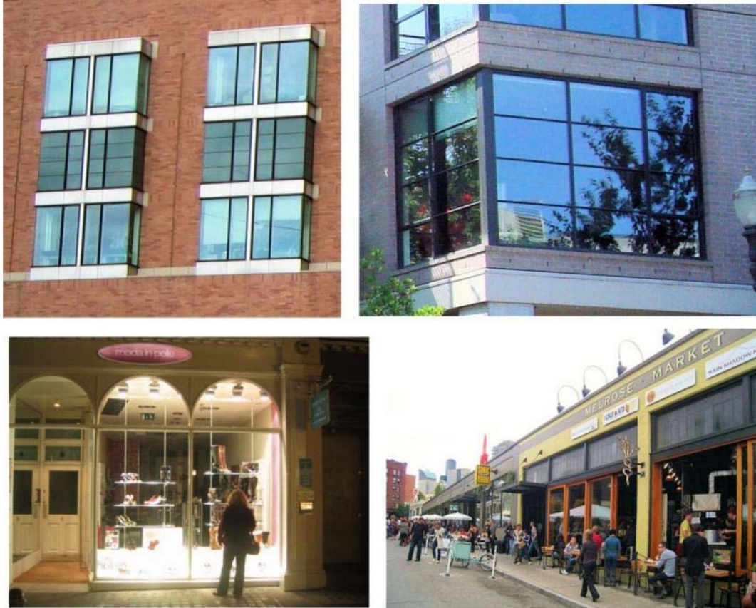
Figure 18.120.040.E.2.b Examples of special window treatments. Note transom windows in the Melrose Market façade.
