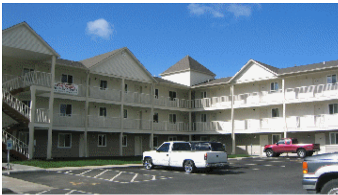
Figure 18.120.020.C.2.b. Elevated external walkways such as this are not allowed
