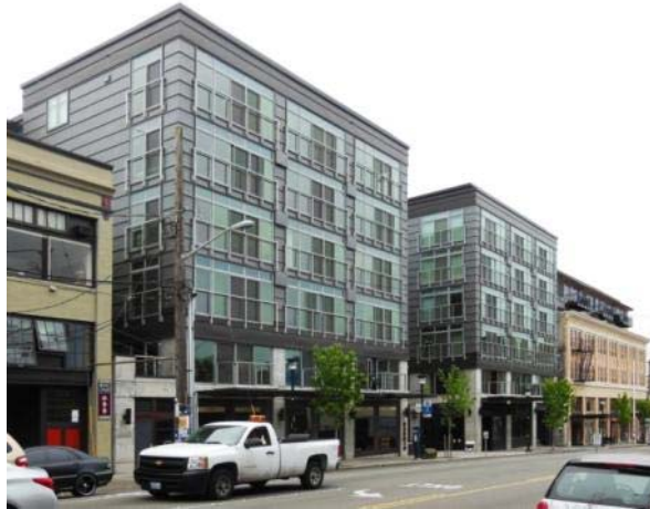
Figure 18.120.040.D.2.c Example of vertical indentation to visually break up the scale of a large building.
