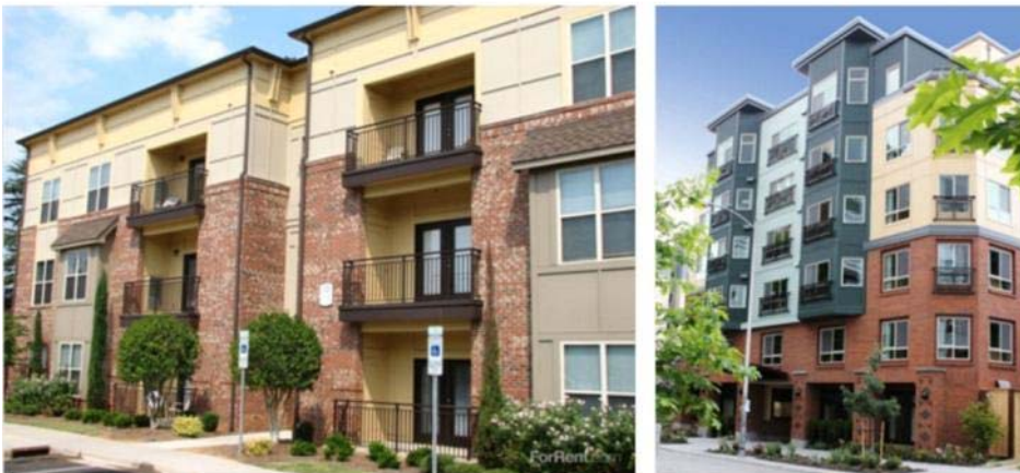
Figure 18.120.040.D.2.b. Examples of articulation of residential building facades. All examples use window fenestration and vertical building modulation elements. The upper examples use a mixture of material changes and detail components to further articulate the façades. In the lower left example, the balcony element’s dramatic mix of color, material and projection are effective in meeting the standards. The lower right example adds a combination of material and color changes and building modulation to help meet the standards.
