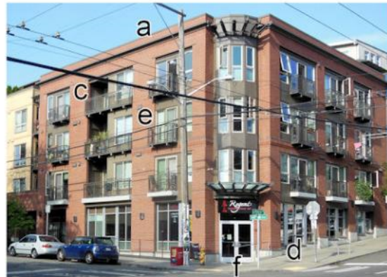
A new traditionally styled building
