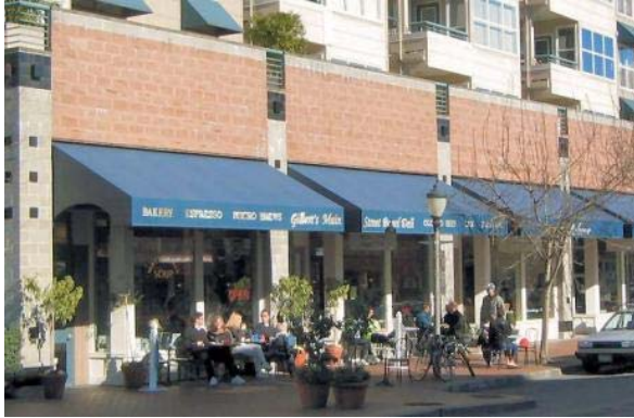
Figure 18.120.040.G.2.b. The above façade illustrates an acceptable alternative example, as CMU is used as the primary cladding material. Note the use of split-façade CMU's above each of the awnings and coupled with the use of smooth-façade CMU's on the vertical columns (which employ black accent tiles for added interest).
