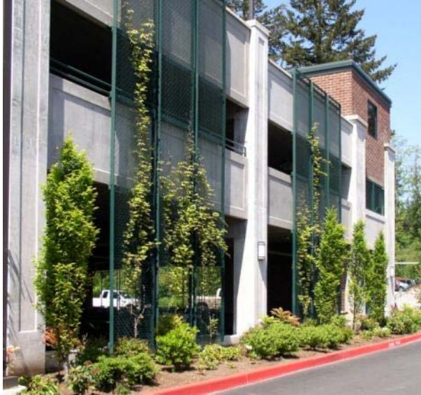
Figure 18.120.040.I.2.a The side of this parking garage includes decorative grillwork, and a raised brick planter to enhance the pedestrian environment.
