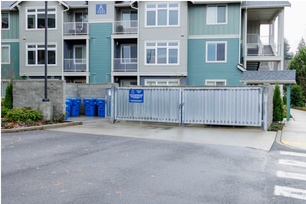
Figure 6 Multi-Family Collection Site
