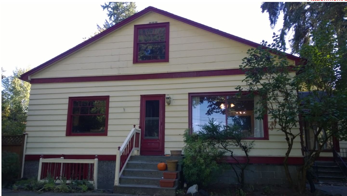
Figure 11: Rear (East) Elevation (September 14, 2016)
