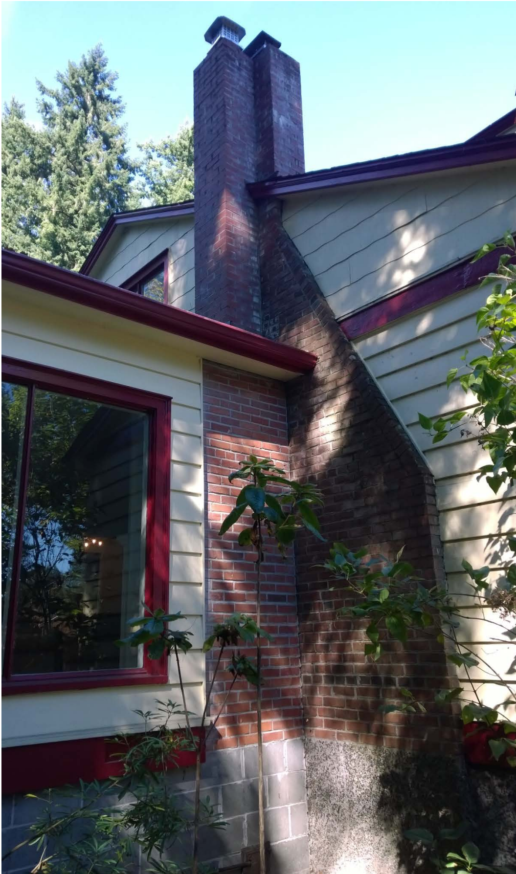
Figure 15: North Addition Juncture (September 14, 2016)
