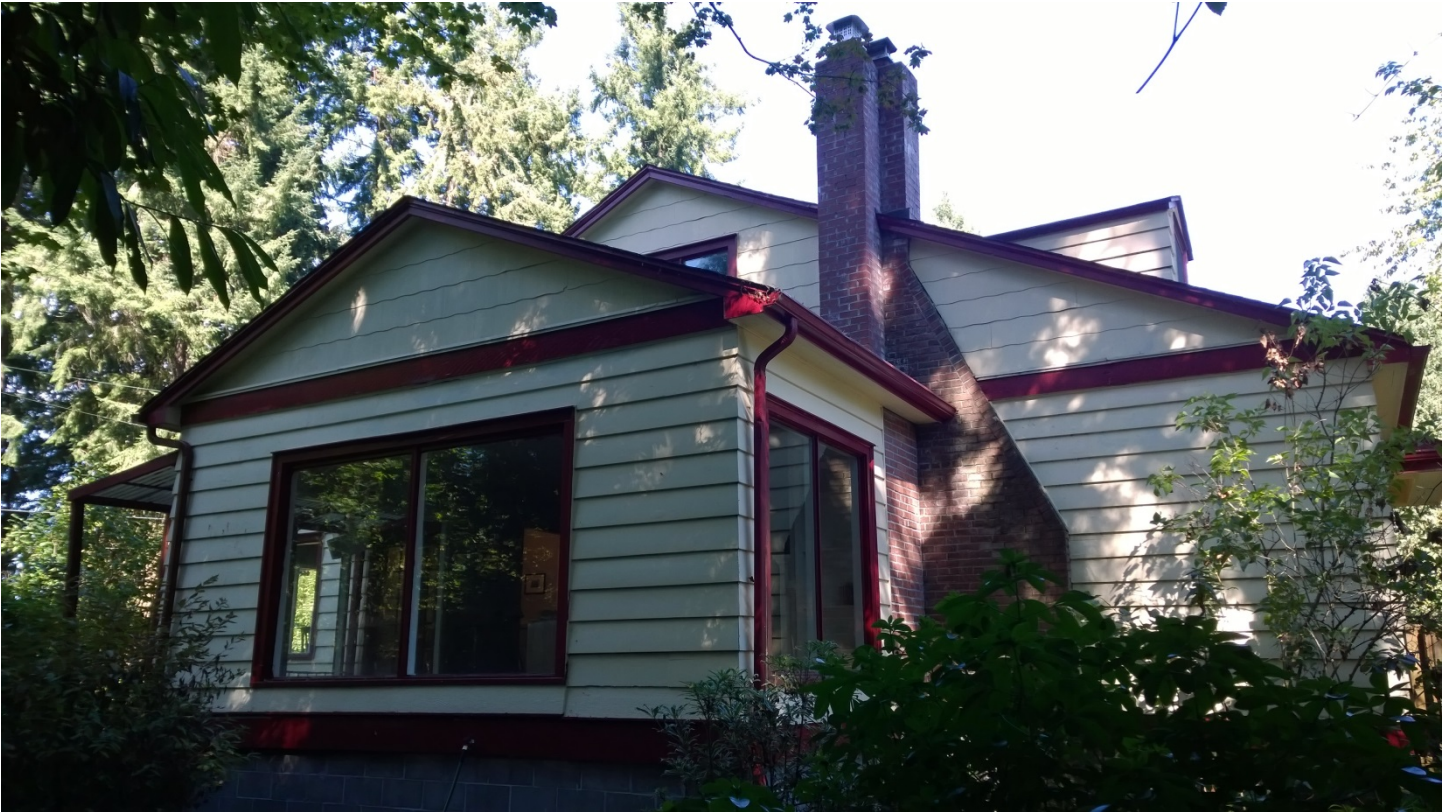
Figure 9: Side (North) Elevation – Facing Southeast (September 14, 2016)
