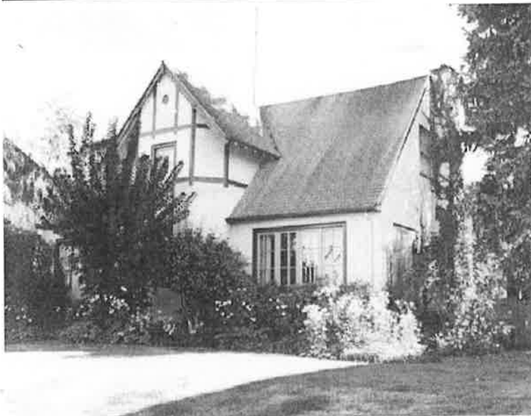
View of northwest corner taken 9/27/1985 Photography Neg. No. (Roll No./Frame No.): 21-24A Comments:
