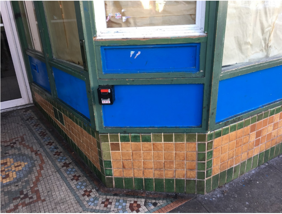
Entry windows rehabilitated
