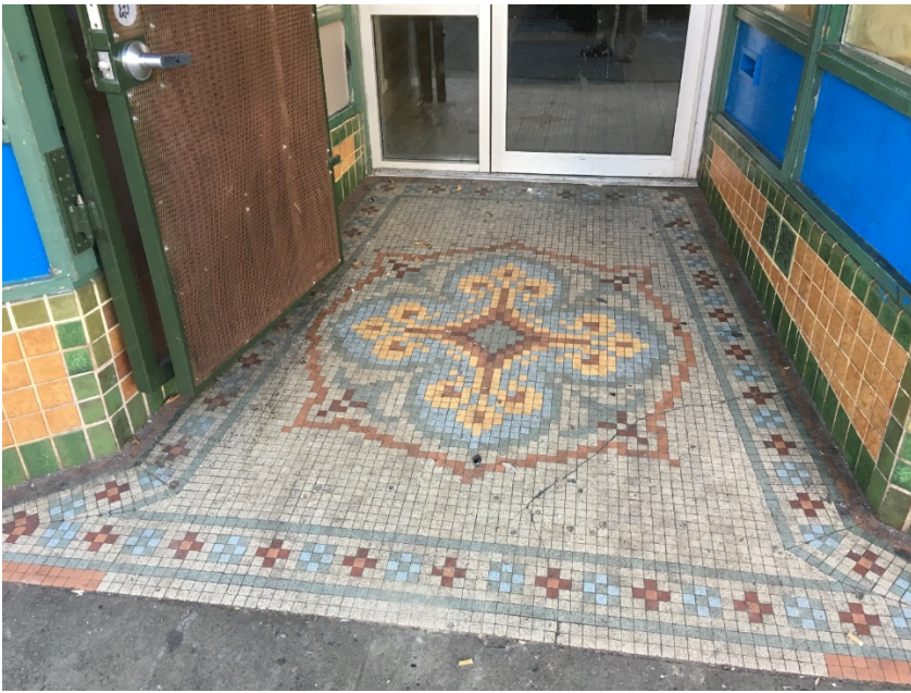
Entry, before and after. Tile photos have been preserved.
