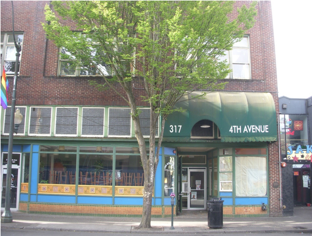
Façade, Before and After
