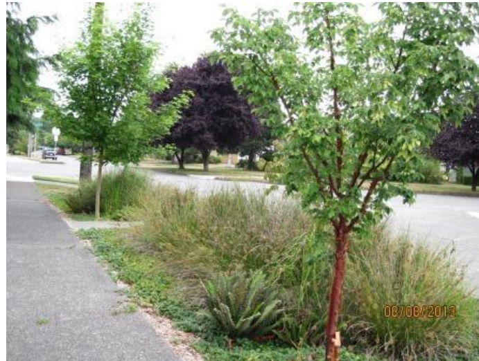
Figure 1 - Bioretention Area installed on existing landscape strip to treat roadway runoff
