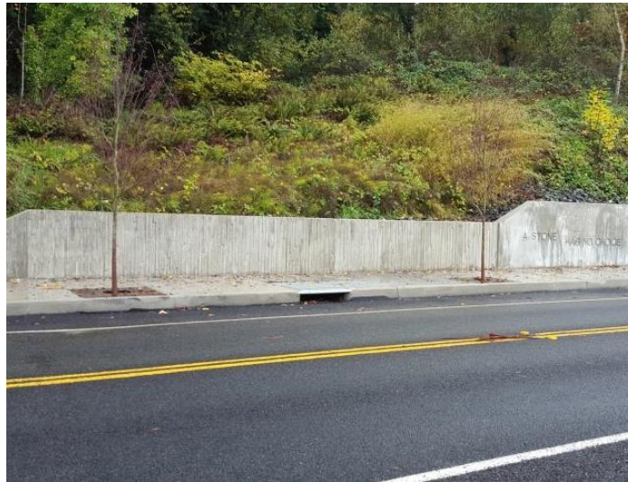
Figure 6 - Modular Wetland System (MWS)® installed on West Bay Drive
