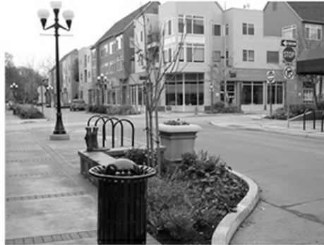
Bulbout (narrows crossing distance for pedestrians and slows traffic)
