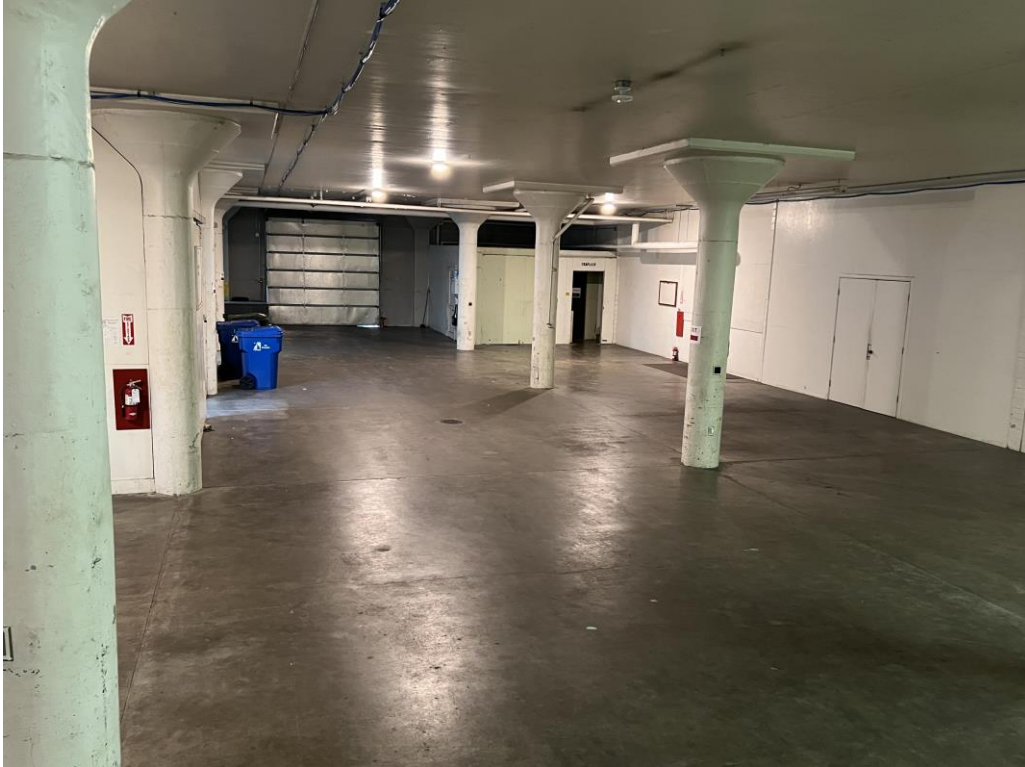
14 of 22 (WA_Thurston_NationalGuardArmoryOlympia_0010) View of basement garage area looking west.
