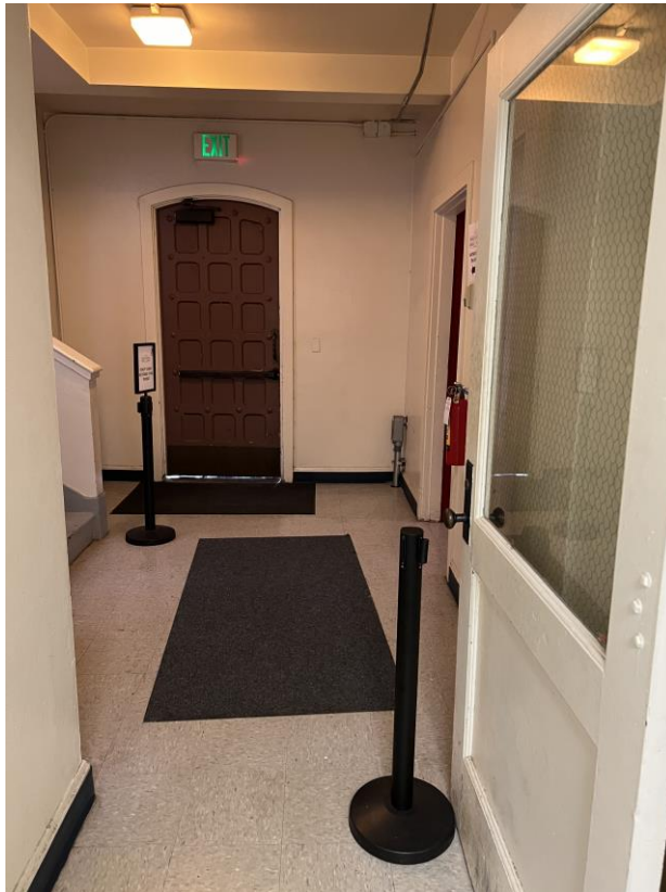
7 of 22 (WA_Thurston_NationalGuardArmoryOlympia_0005) View of the secondary entry, northeast corner.
