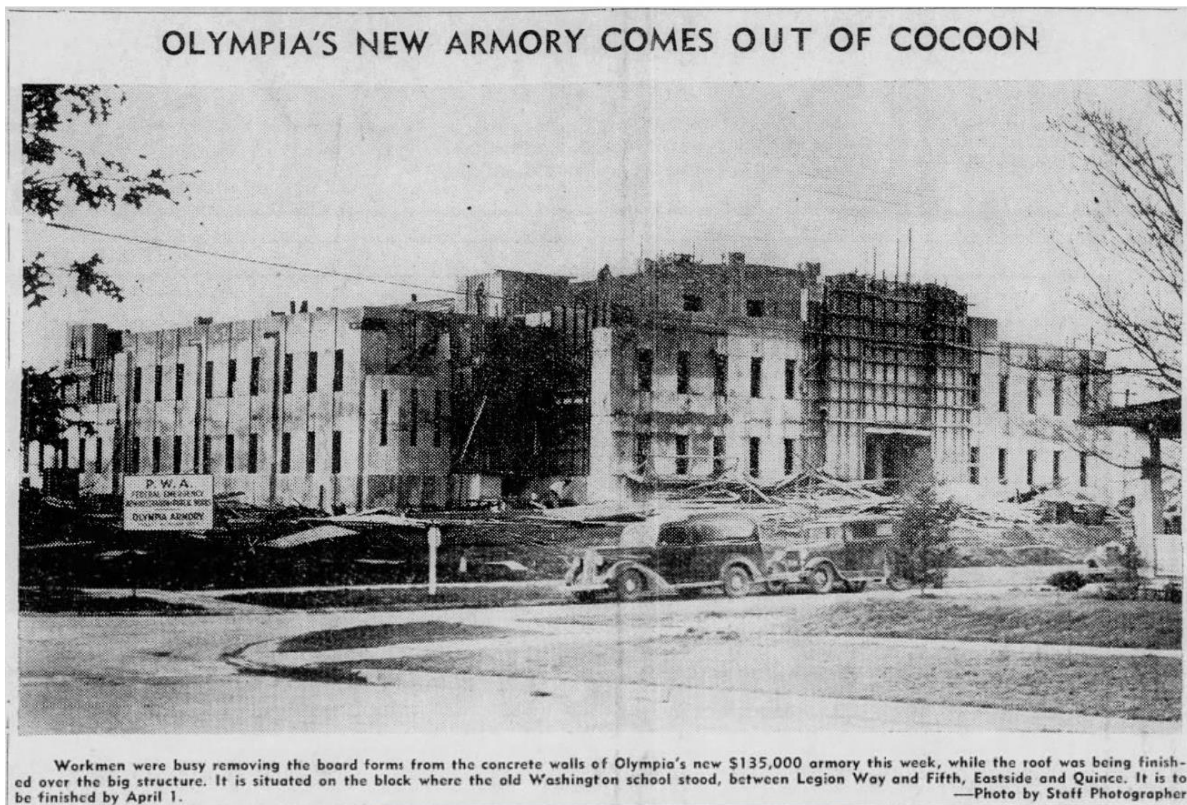
Construction Image – The Olympian – January 24, 1939.
