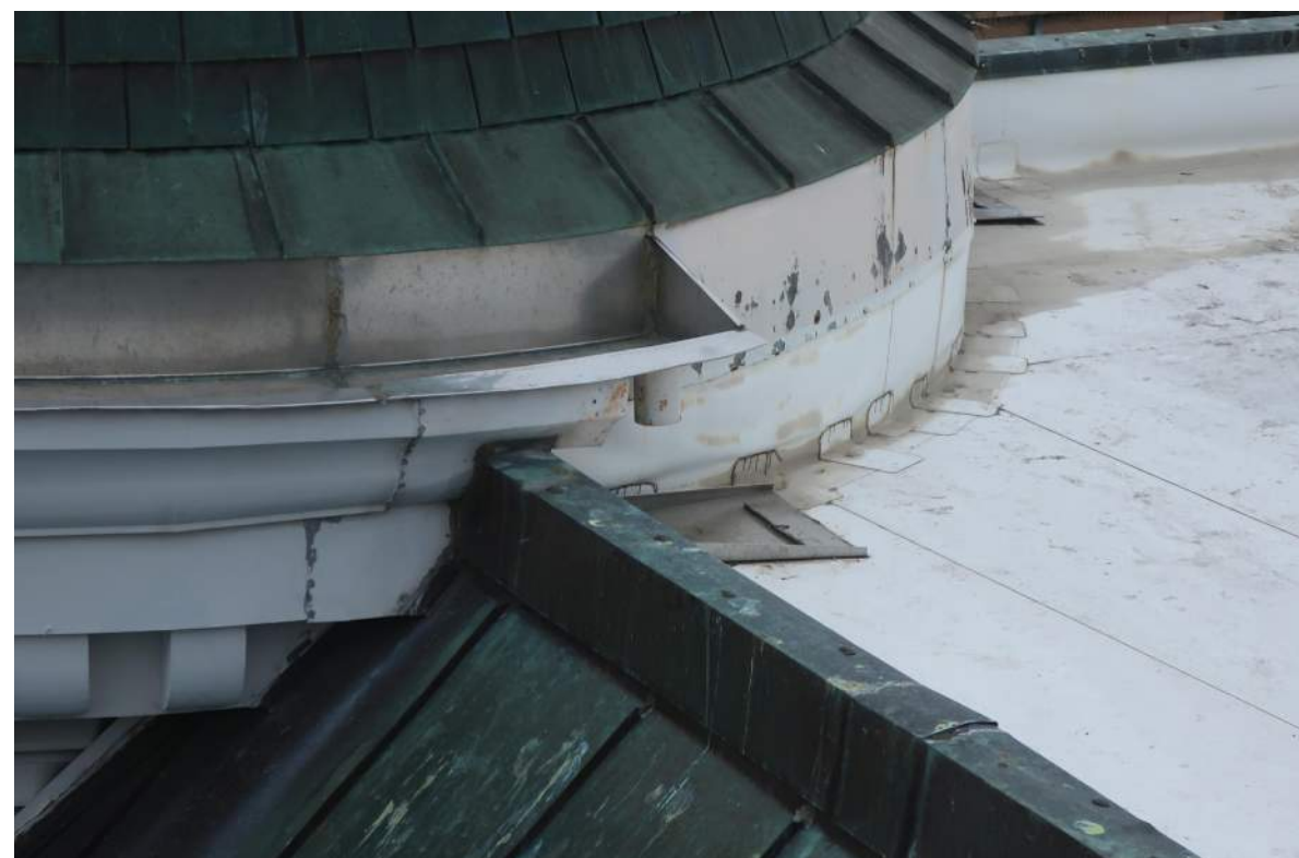
15 BASE OF TURRET AT LOW-SLOPE ROOF ON BUILDING 'B'
