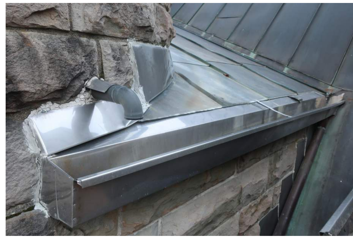
3 S.S. INTEGRAL GUTTER AND STEP FLASHING
