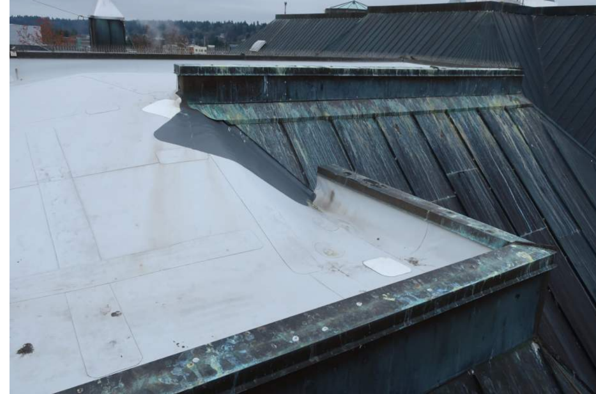
7 BUILDING 'A' LOW-SLOPE SINGLE-PLY ROOFING AND COPPER COPING
