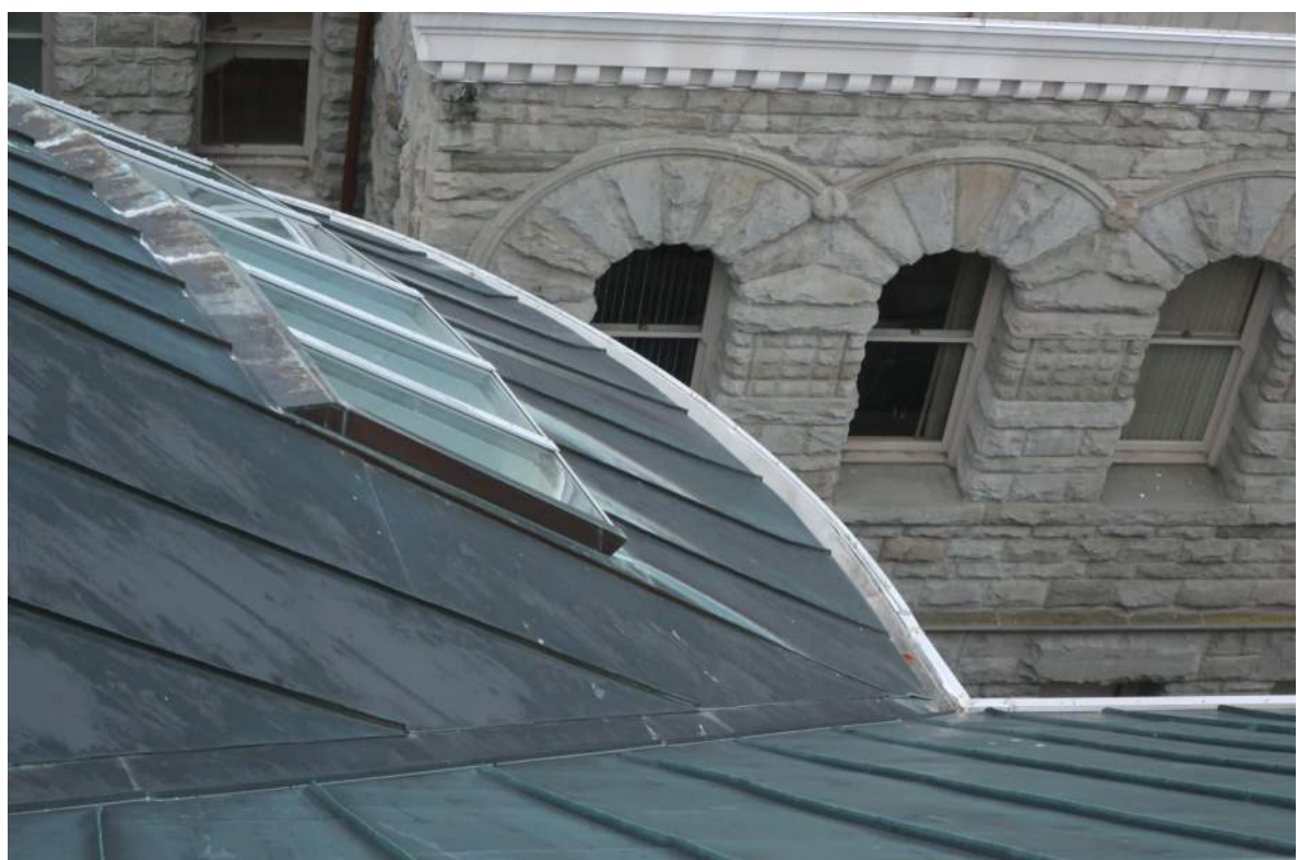
12 BUILDING 'B' NORTH SKYLIGHT
