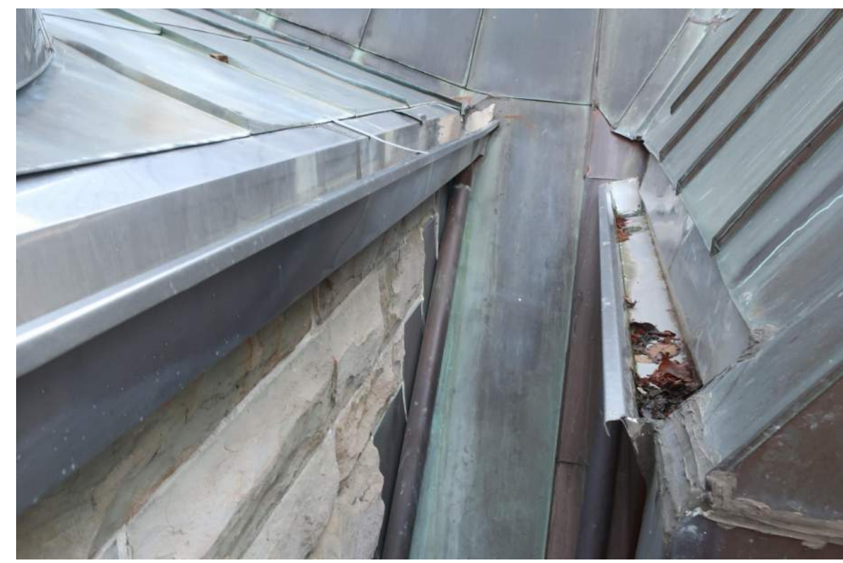
5 SIDEWALL STEP FLASHING AND S.S. GUTTER
