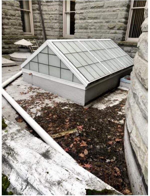
9 GARAGE ROOF SKYLIGHT AND DOWNSPOUT
