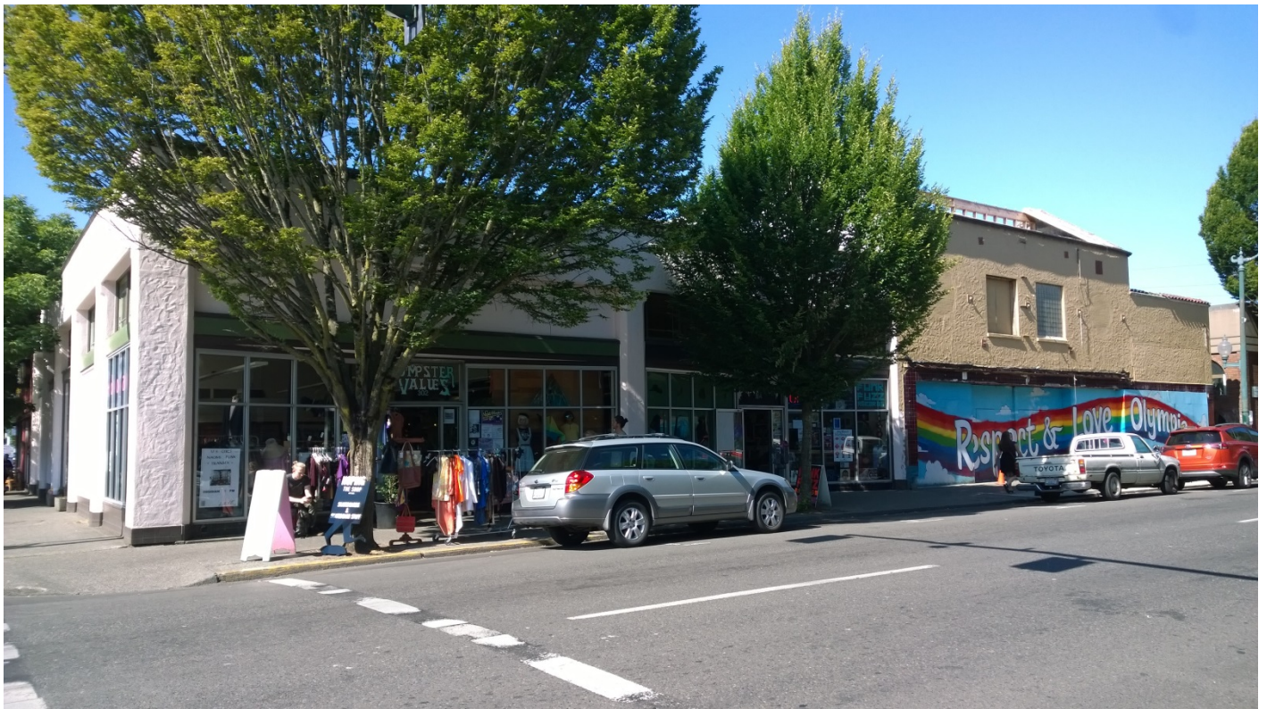
Figure 16: South Elevation with Former Avalon Theater on Right (June 29, 2016)
