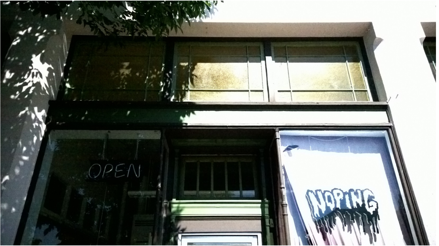
Figure 20: Storefront Detail – West Elevation (June 29, 2016)
