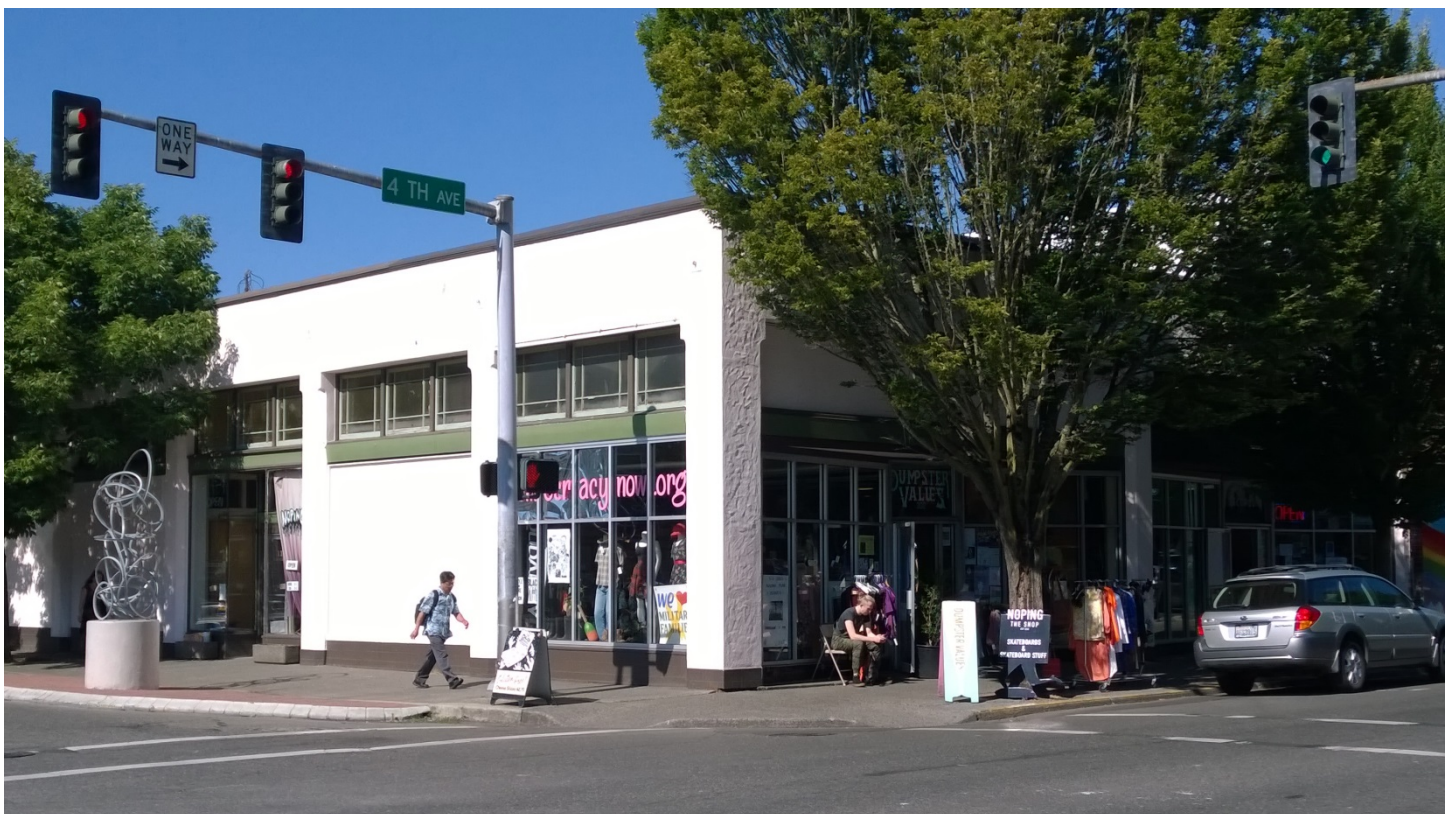
Figure 17: West & South Elevations (June 29, 2016)
