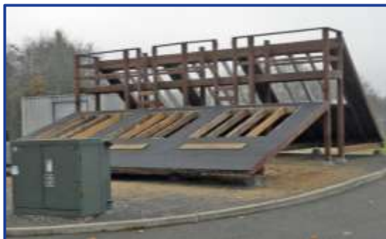
Figure 120: Roof Props at the OFD Training Center
