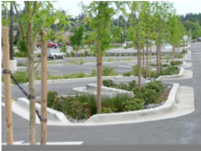
Concave landscape islands can serve dual purposes: visual relief and stormwater infiltration (Element 12).
