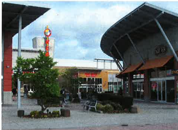
Renton Landing: MAKERS' planning concept (top) led to the completed development (above).
