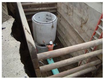
Installing a deep sewer <u>maintenance hole</u> manhole on Henderson Boulevard as part of a planned capital improvement project.
