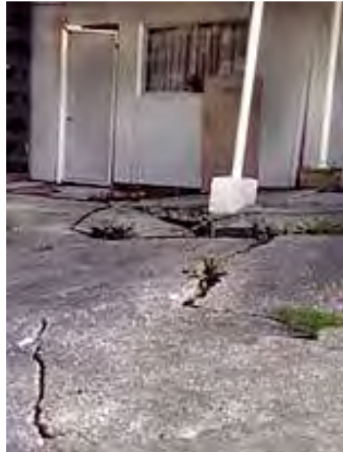
Figure 63: Photo of Carlyon Beach property damaged by the '98-'99 winter landslides. Source: Slaughter, 2016
