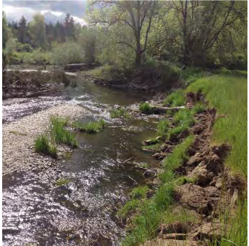
Figure 19: Fast-moving water removed riparian vegetation along a rural stretch of the Deschutes River during the winter of 2015-'16, making the streambank vulnerable to erosion. Source: TRPC
