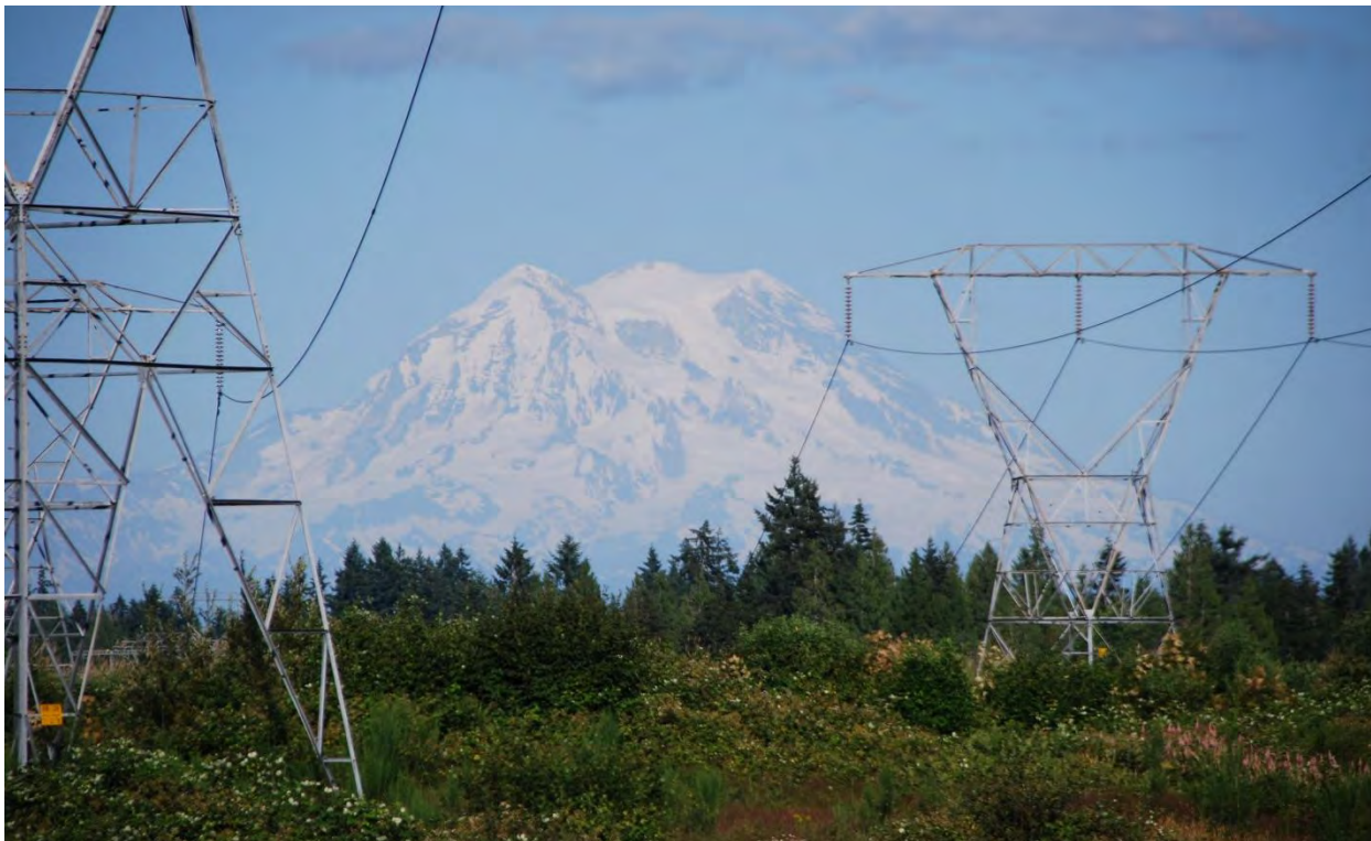
Figure 25. Mount Rainer looms over transmission lines in Thurston County, where Puget Sound Energy has about 120,000 electric customers. Source: TRPC
