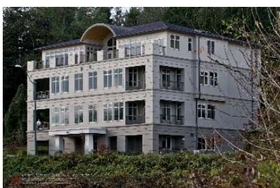
Baywood Building, Olympia, WA Mixed-Use Condominium, 2012
