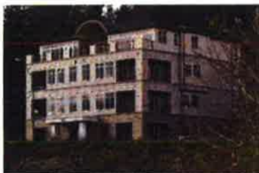
Baywood Building, Olympia, WA Mixed-Use Condominium, 2012
