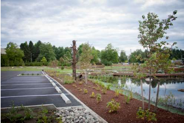
Porous pavement, bioretention, and constructed wetlands demonstrate stormwater options for low-impact development at Yauger Park.
