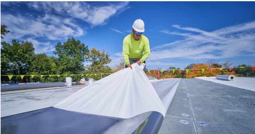
Single Ply TPO Roof
