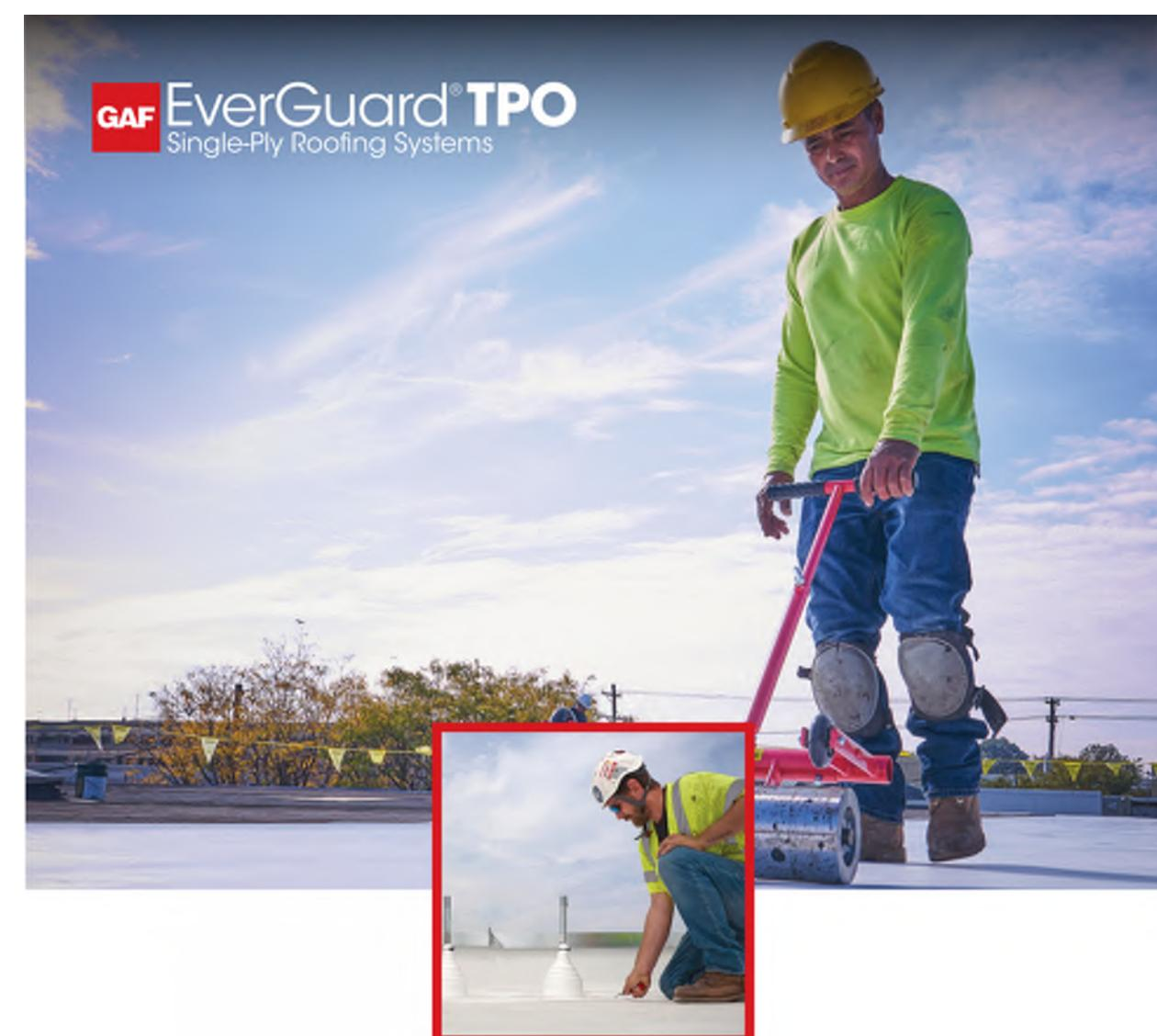
TPO (thermoplastic polyolefin) is a single-ply roofing membrane that offers excellent performance and has been the most popular roofing membrane for many years. GAF
