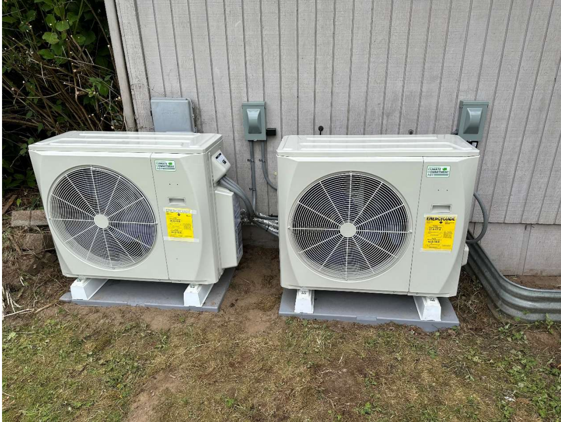
Heat pump outdoor units installed at a home in Olympia.
