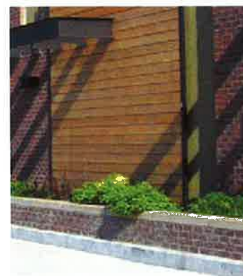
Building detailing & raised planter
