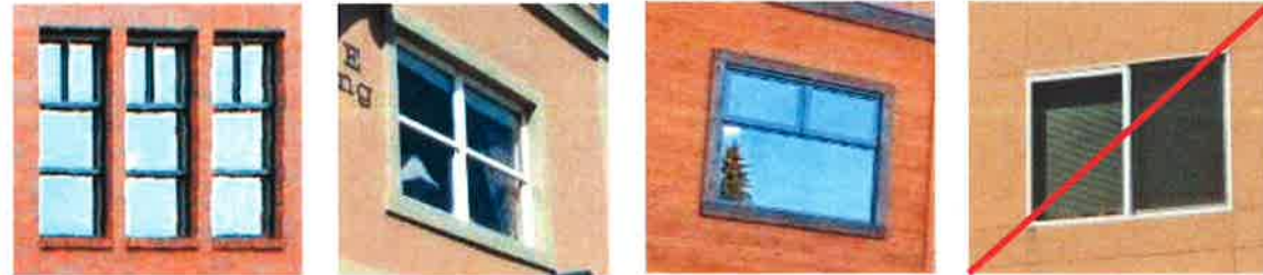
Acceptable and unacceptable (far right image) window design on upper floors. Note the windows in the brick building on the left are recessed from the facade. The windows in the middle images include trim. The image on the right includes no trim or recess/projection, and thus would not be permitted.
