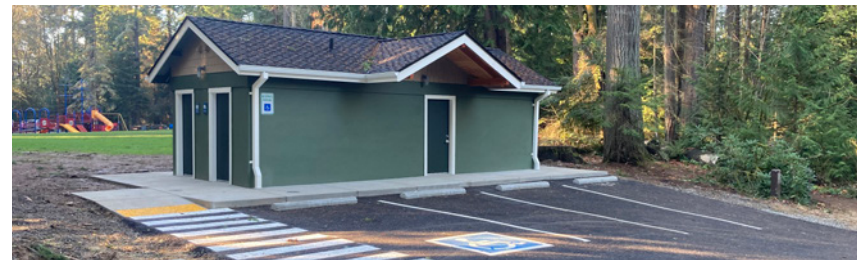
ADA Upgrades to Restroom #2 at Priest Point Park.
