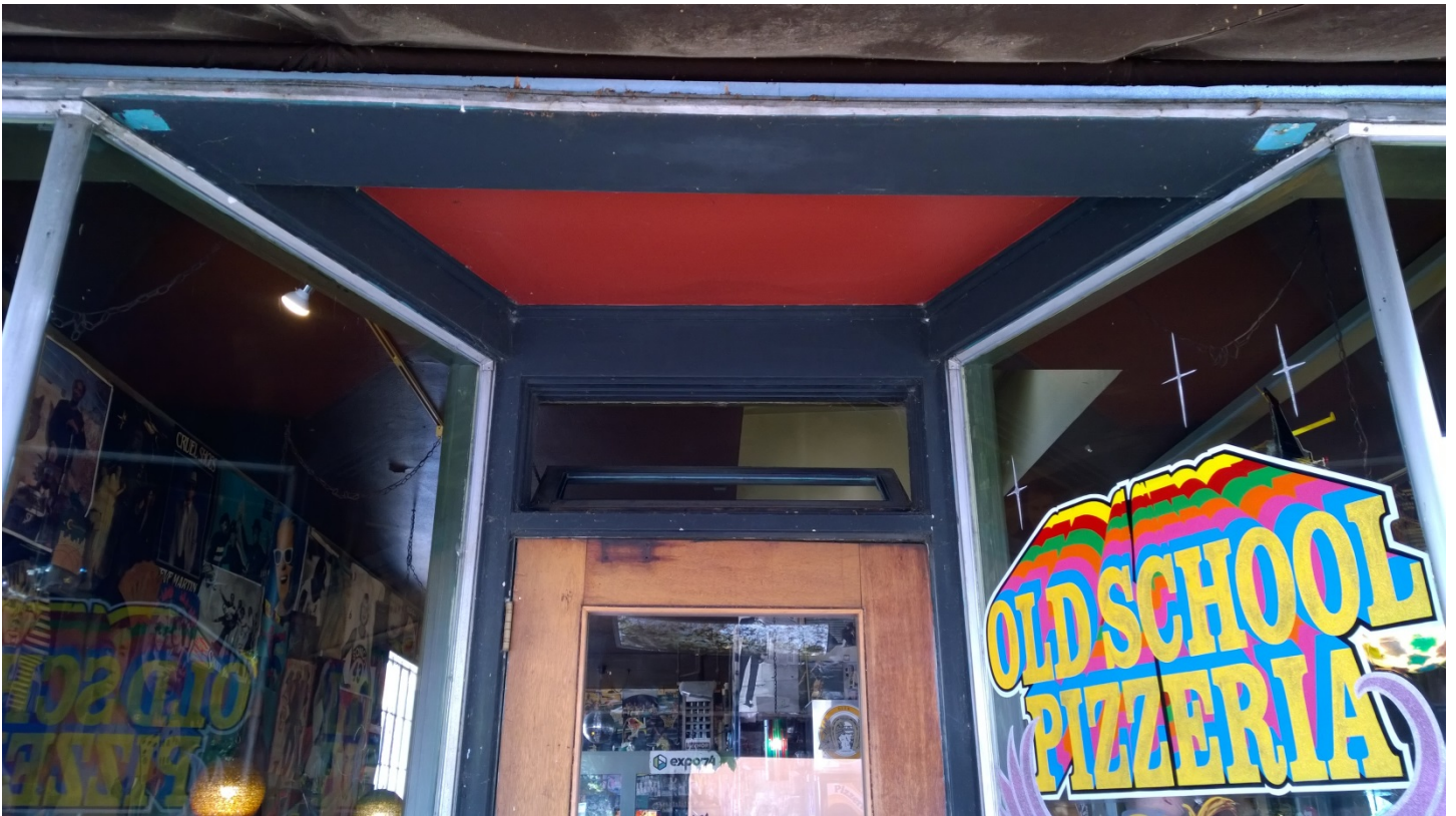
Figure 15: Front Entrance Detail
