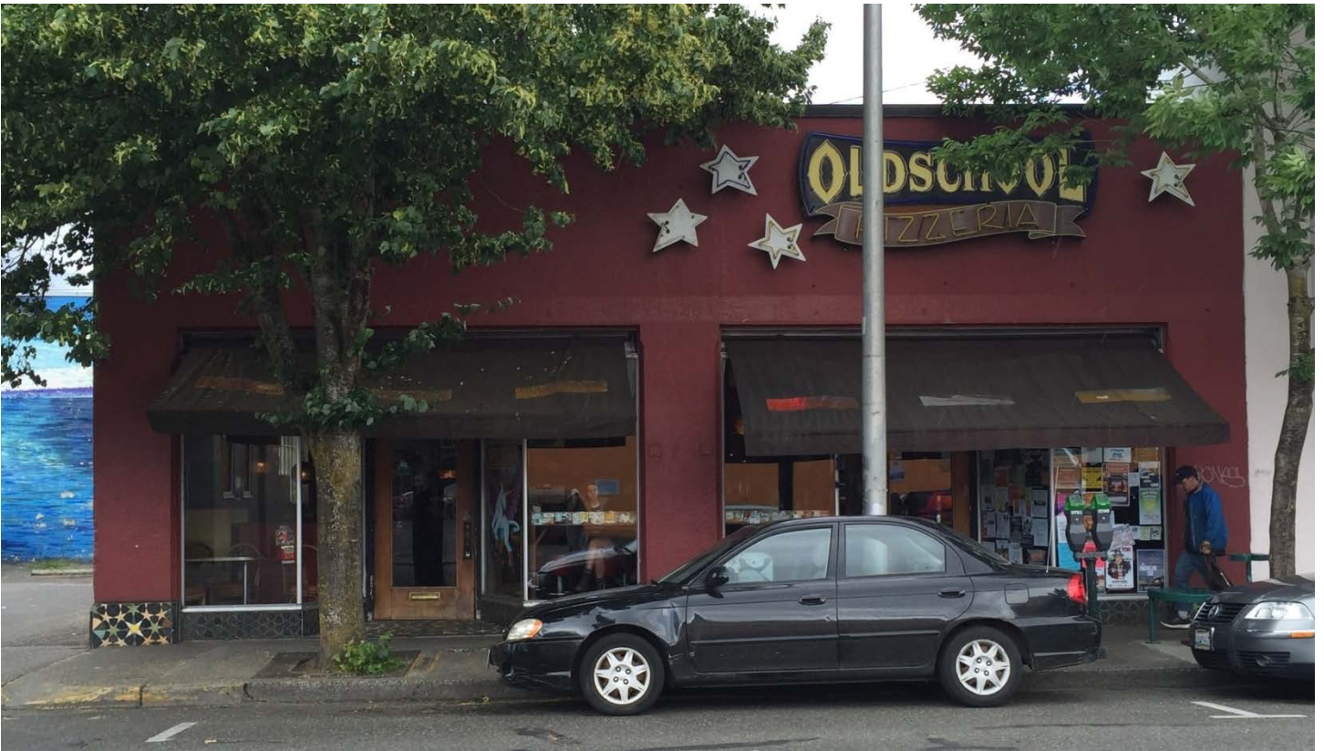
Figure 18: Front (West) Elevation (facing east)
