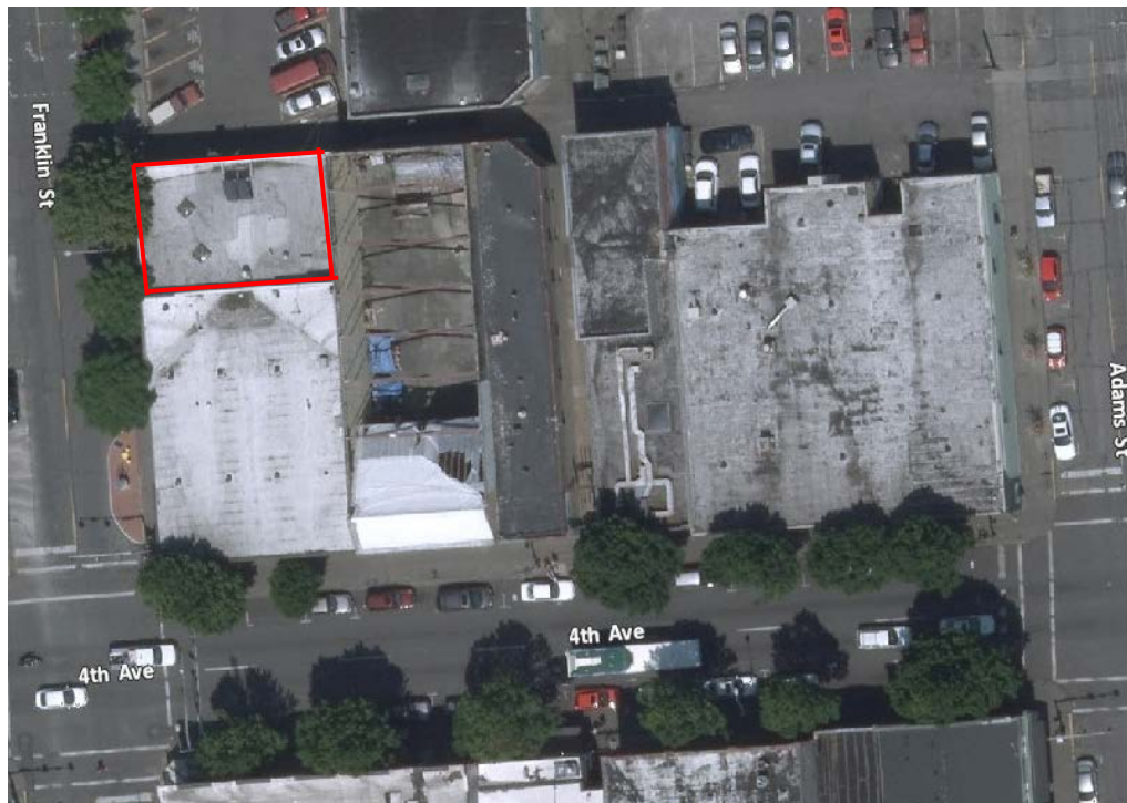
Figure 1: 2015 aerial photo showing building, Olympia Online Mapping.
