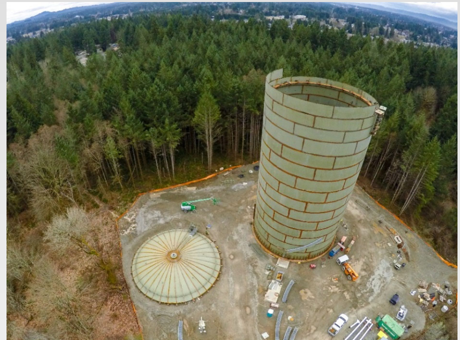
LBA Reservoir Construction (formerly known as Log Cabin Reservoir)
