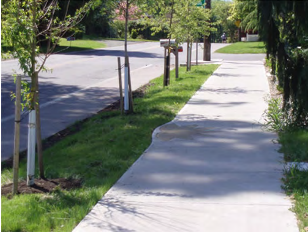
A new sidewalk is buffered by a planter strip and street trees on San Francisco Avenue.
