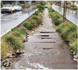
C Green stormwater infrastructure
