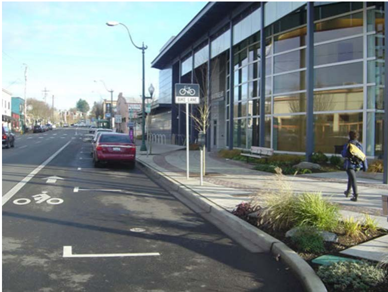
4th Avenue near City Hall redesigned with bike lanes and wider sidewalks [[Photo: 4thAveCityHallBikeLanes.jpg align=right caption=4 th Avenue near City Hall redesigned with bike lanes and wider sidewalks.]]
