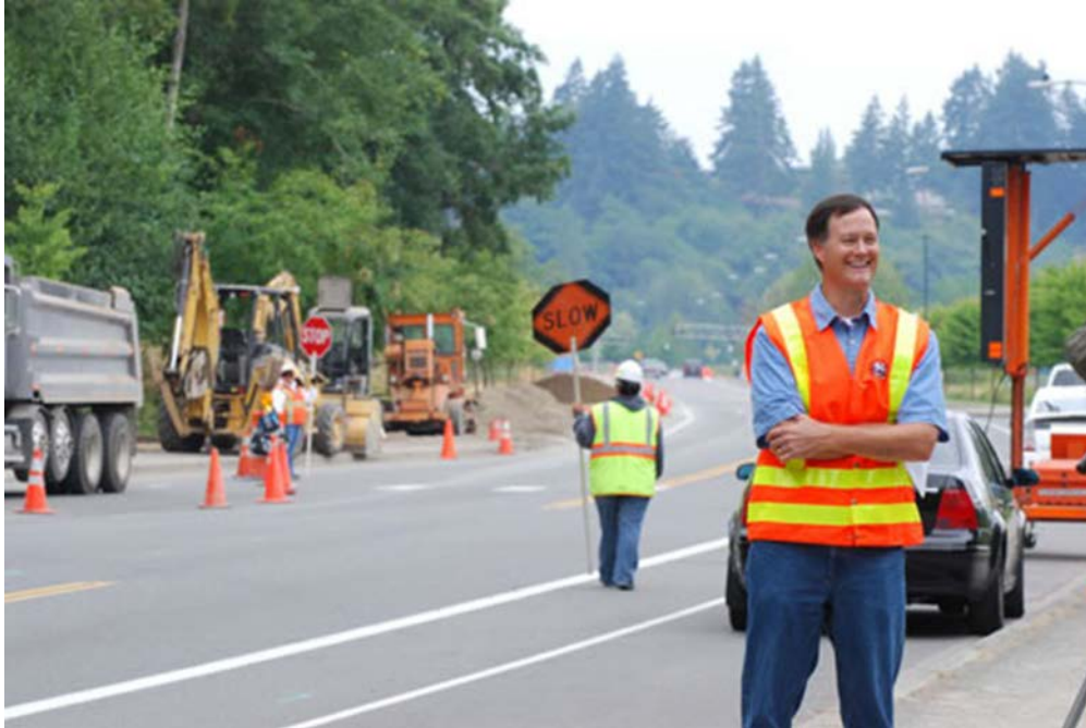
RW Johnson Boulevard is rebuilt
