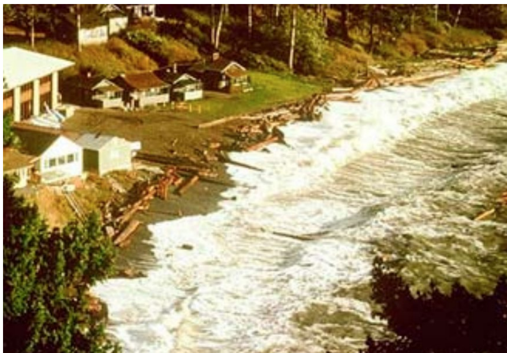
Figure 3-2: Example of high tide windstorm causing significant beach and backshore change at Rosario Resort in San Juan County (Johannessen and MacLennan 2007)
