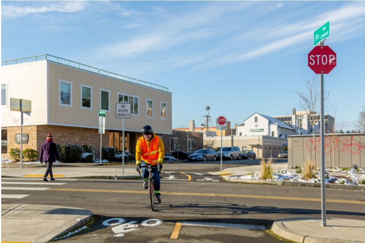
A bicycle-only crossing on 7th Avenue at Jefferson Street, which also includes a marked crosswalk for pedestrians with ADA compliant curb ramps.
