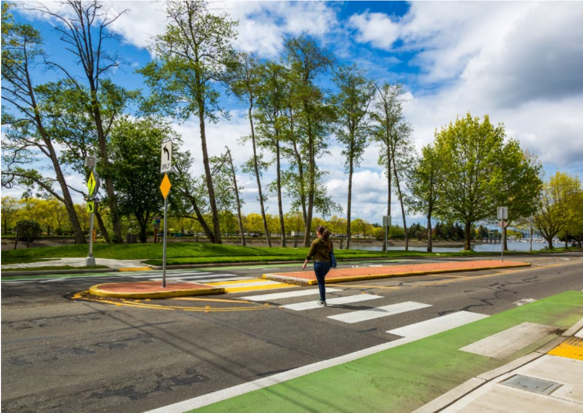
The flashing beacons, island, and crosswalk marking make crossing East Bay Drive at Olympia Avenue safer and more inviting.
