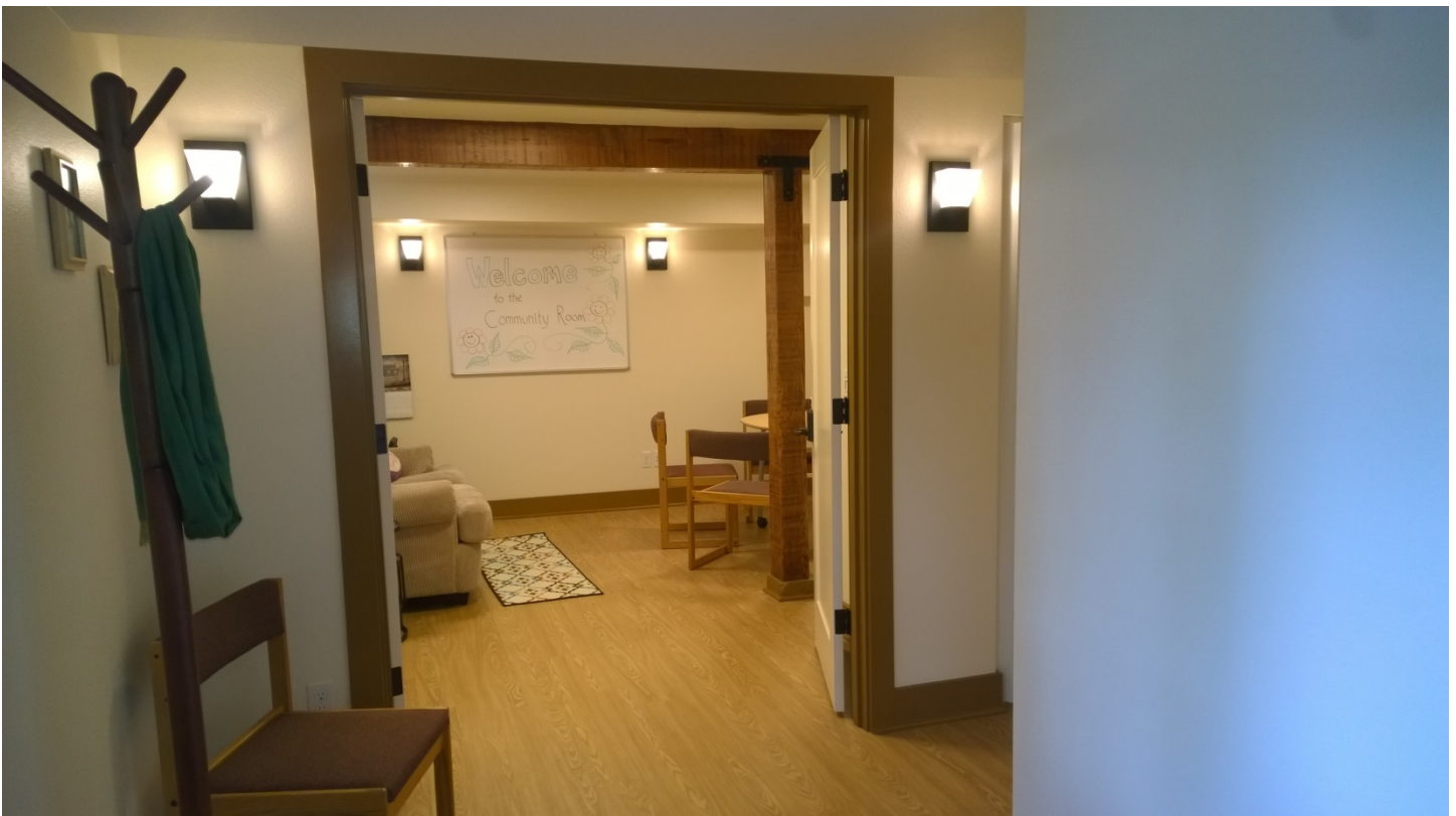
Figure 13: The previously unfinished basement was entirely framed out to create accessible meeting and treatment spaces. This is the view from the entrance into the main meeting and treatment room.
