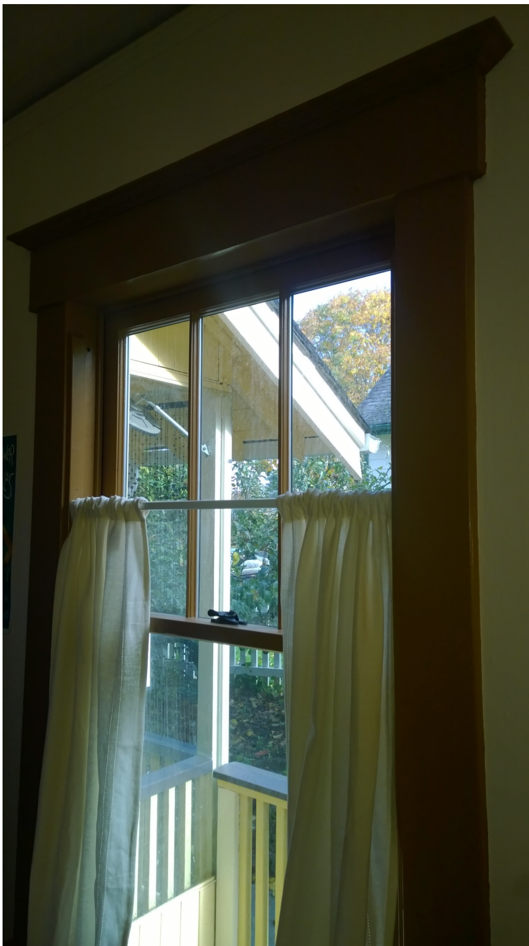
Figure 10: All original windows were refurbished and refitted with double-glazed units.
