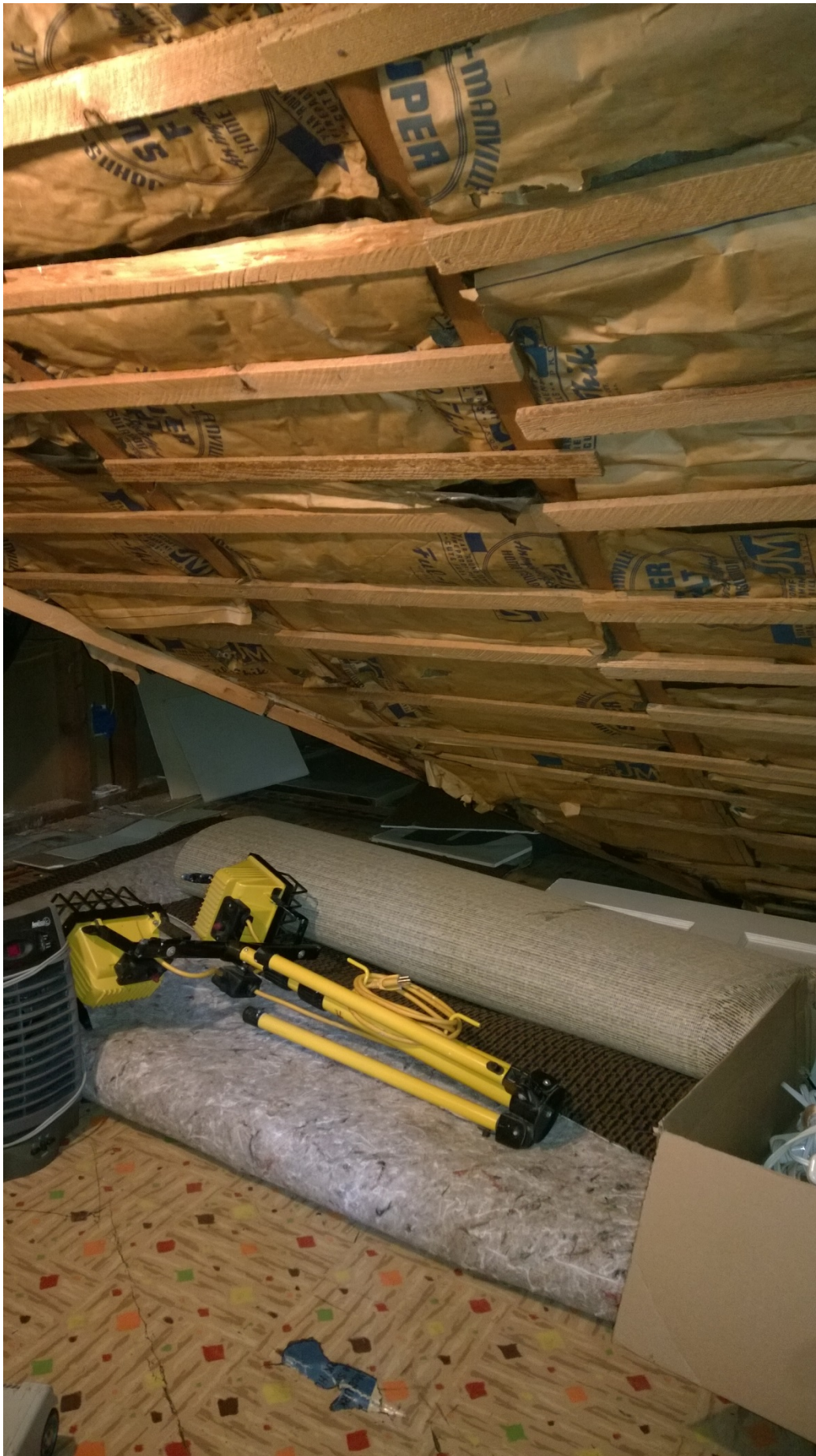
Figure 7: Roof and insulation improvements. Note retention of original or early linoleum.
