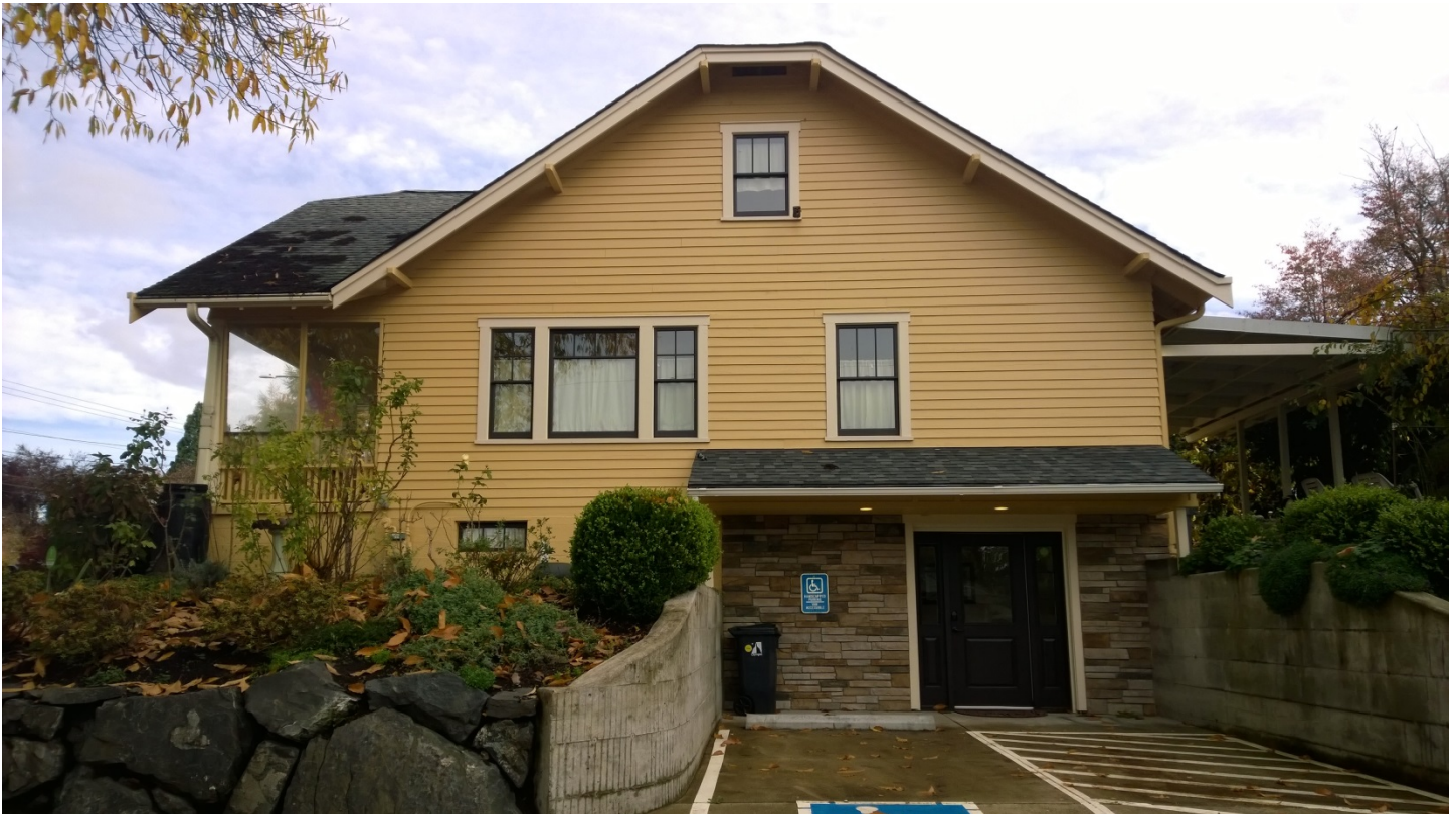
Figure 3: Side (West) Elevation). Note pedestrian entrance alterations to accommodate an accessible entrance and meeting/treatment rooms, replacing a (non-historic) garage door.
