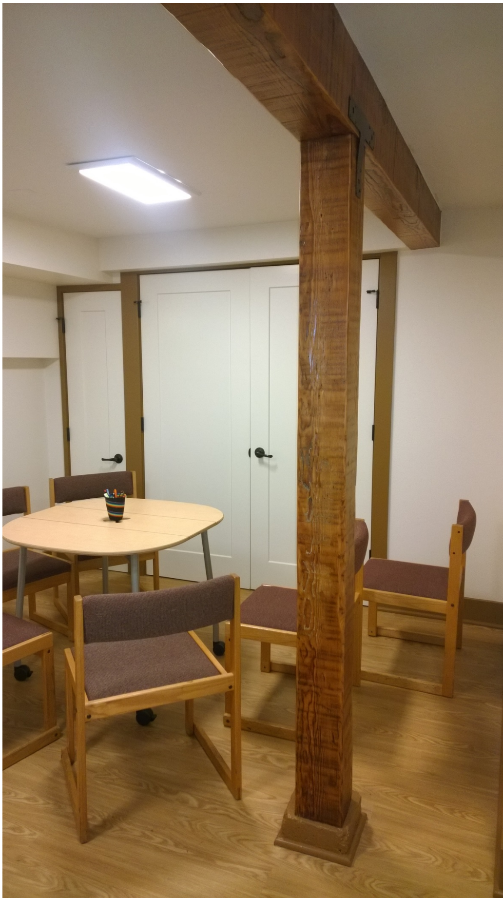
Figure 14: The main accessible meeting and treatment room in the basement. Original framing was retained and is now highlighted as a feature throughout the basement spaces.
