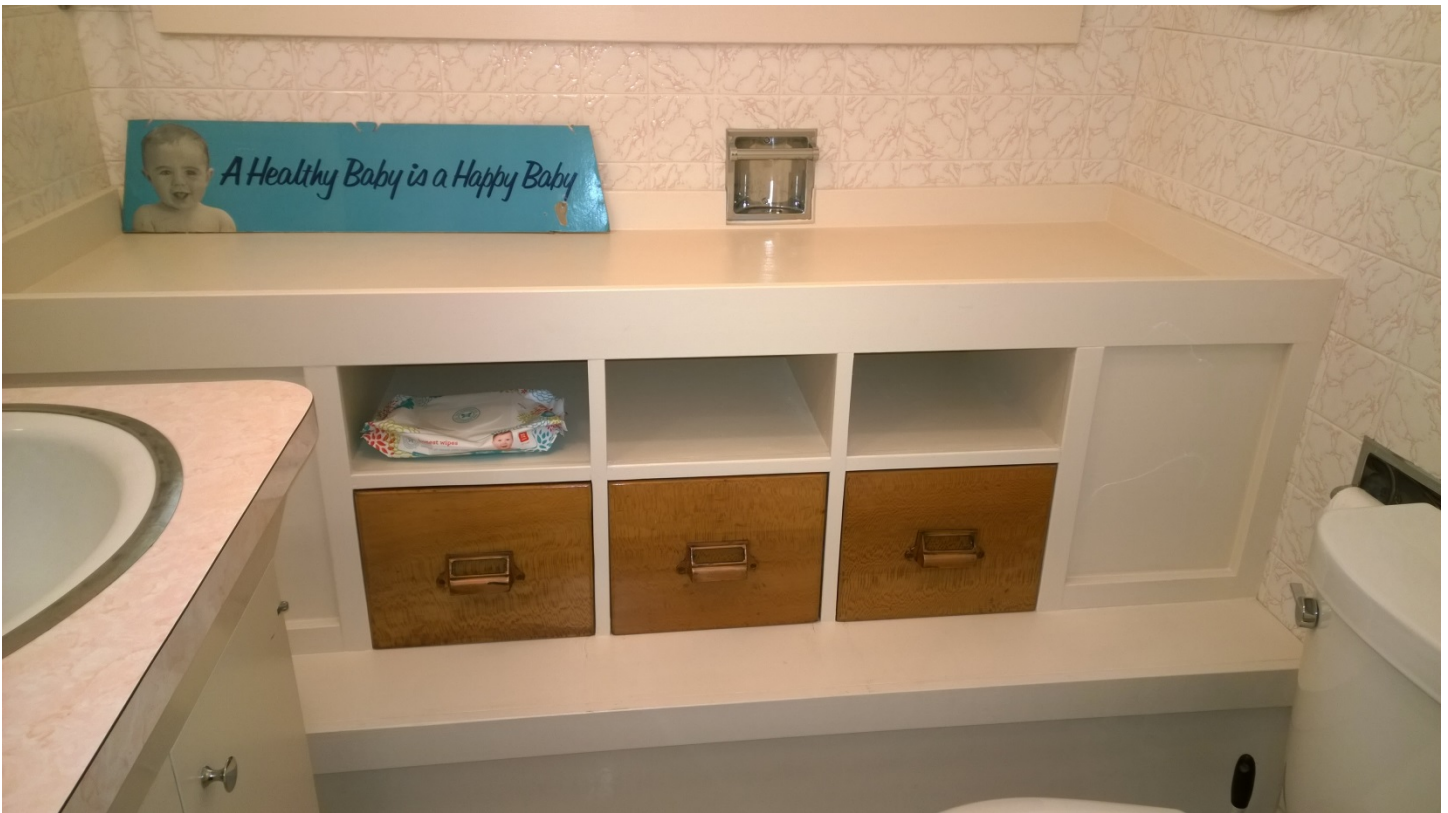
Figure 12: Bathrooms were upgraded while retaining and reusing historic fittings. Here the bath is covered with a baby-changing table that reuses some of the drawers from the pharmacy run by former owners.
