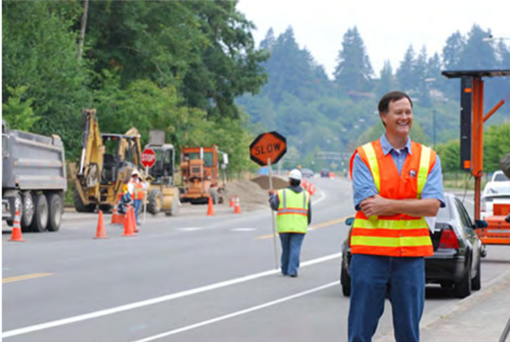
RW Johnson Boulevard is rebuilt.
