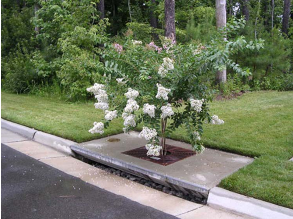
Typical Filterra Bioretention Filtration System curbside installation
