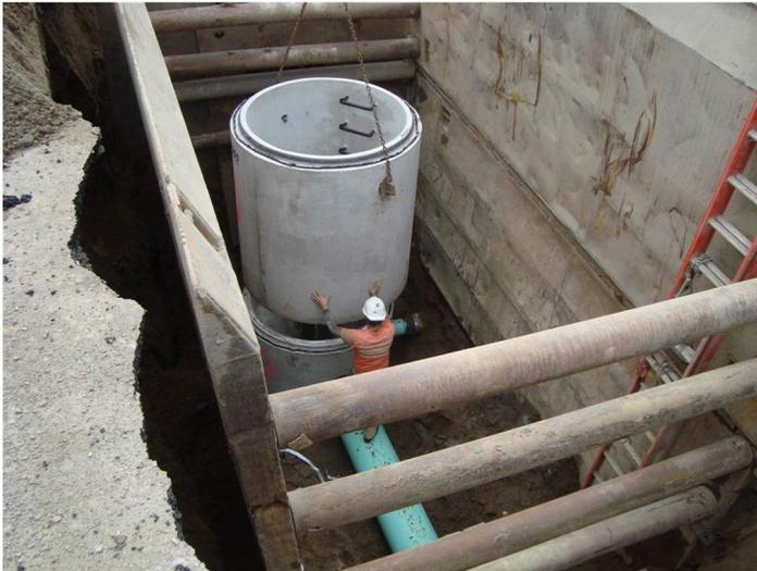
Installing a deep sewer [maintenance hole manhole](#) on Henderson Boulevard as part of a planned capital improvement project.
