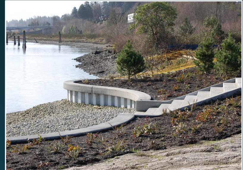
West Bay Park Phase II Cleanup
