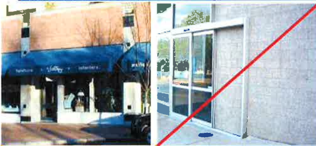
Acceptable and unacceptable concrete block examples. The left example uses a mixture of split-faced colored concrete block and smooth-faced concrete block, together comprising just under 30 percent of the whole façade. The large expanse of smooth-faced concrete block on-the-right above is not acceptable for Briggs Village facades.
