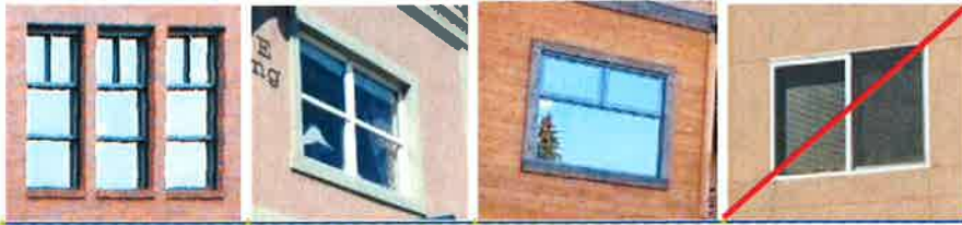
Acceptable and unacceptable (far right image) window design on upper floors. Note that the windows in the brick building on the left are recessed from the façade. The windows in the middle images include trim. The image on the right includes no trim or recess/projection, and thus would not be permitted.
