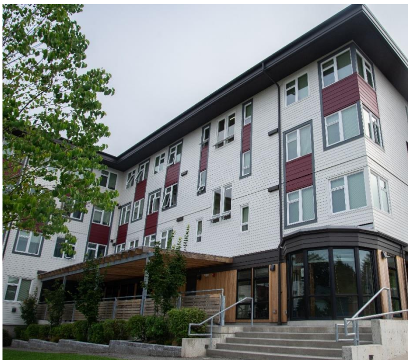
Devoe II Veterans Housing (50 units) typifies the housing goals of the Home Fund
