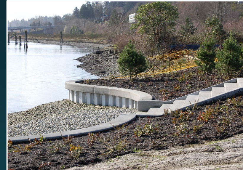
West Bay Park Phase II Cleanup
