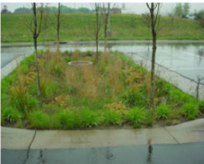
Areas proposed for infiltration need to be protected from compaction and sediment laden runoff during construction.
