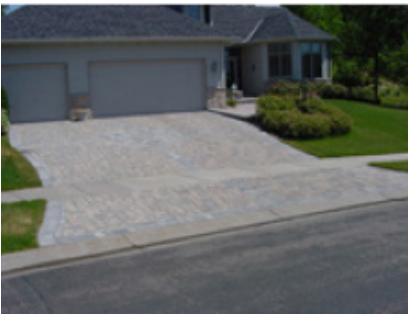
Reducing the impervious surfaces associated with driveways would increase opportunities for infiltration, but any changes to reduce the allowed driveway width from the edge of the street to the garage would also create potential design challenges for homes with wider garages (Element 10).
