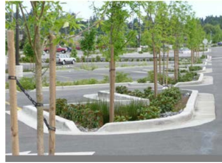
Concave landscape islands can serve dual purposes: visual relief and stormwater infiltration
