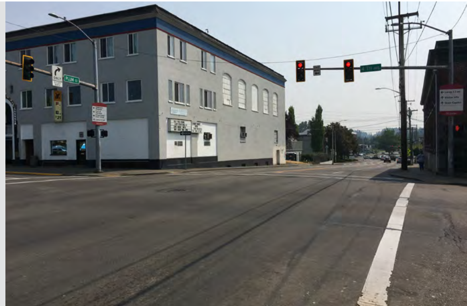
View looking south towards the portable unit at the Salvation Army from the intersection of Plum and State.
