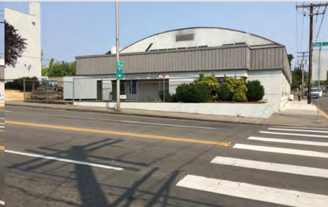
View of portable unit at the Salvation Army from across Plum St.
