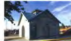
C. - Comfort Station, Percival Landing West
