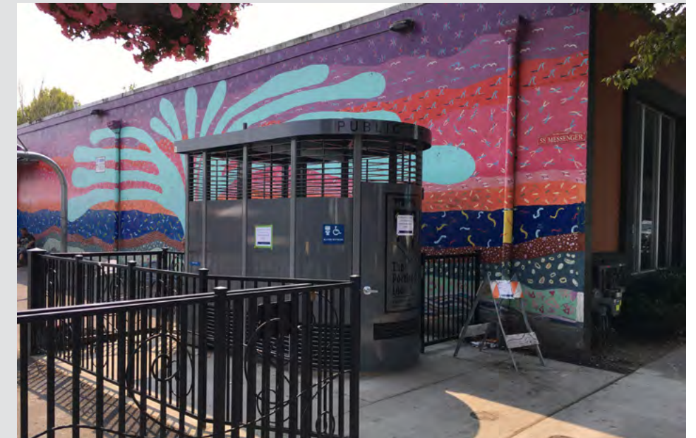
The Portland Loo at the Artesian Commons.
