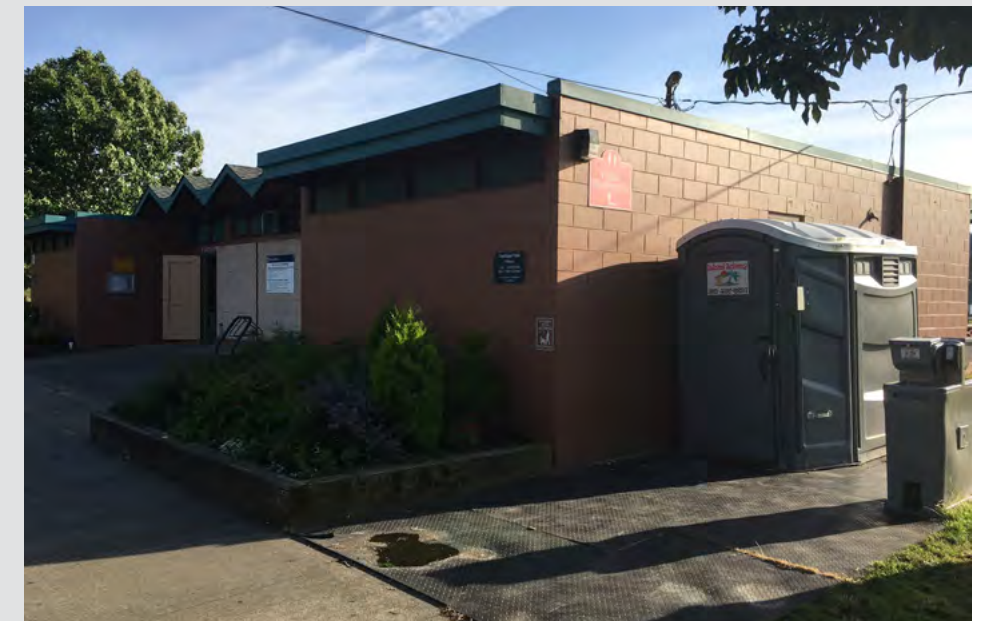
Hand washing station next to the portable unit at Heritage Park Bath House.
