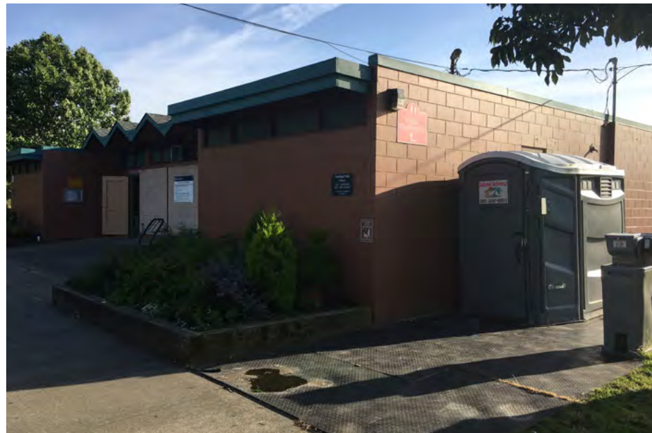
Portable unit at Heritage Park Bathhouse Hours: 24-hours, 7 days a week
