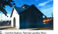
C. - Comfort Station, Percival Landing West
