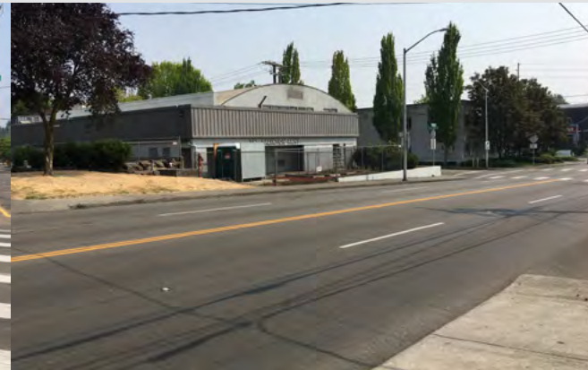
View of Plum St looking south towards the portable unit at the Salvation Army.
