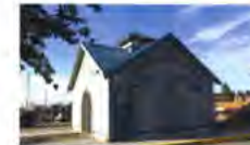
C. - Comfort Station, Percival Landing West
