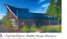
D. - Comfort Station, Shelter House, Showers, Harbor House, Percival Landing
