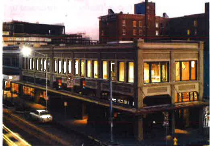
MSGs offices in the Walker Building, Downtown Olympia
