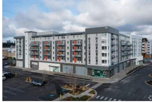
Avalon Alderwood Place 18602 Alderwood Mall Parkway 328 Units; Built 2021
