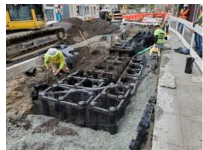
Figure 4-3. New technologies like soil cells allow for proper soil volumes for urban trees while still accommodating utilities, irrigation, and paving in tight conditions. Source: Seattle Department of Transportation
