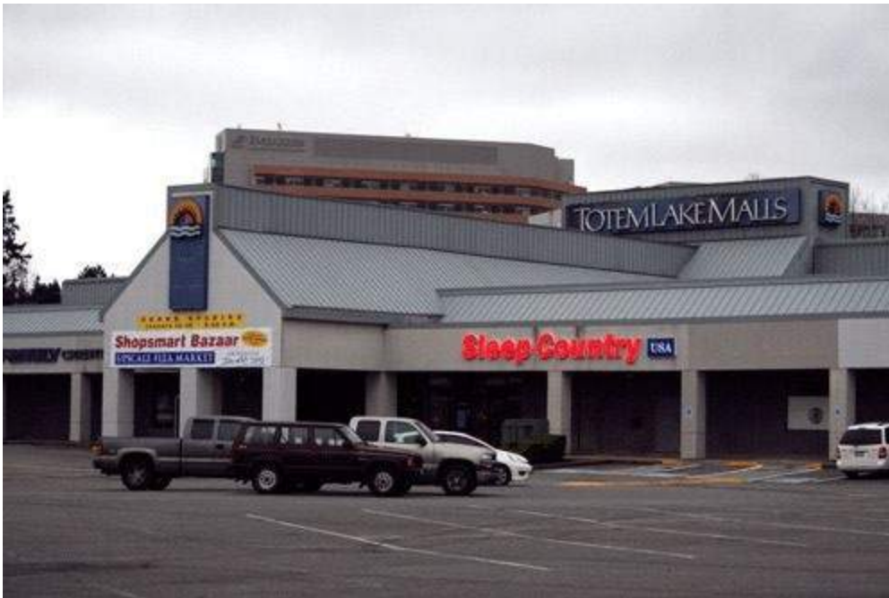
Figure 102. Totem Lake Mall Prior to Redevelopment
