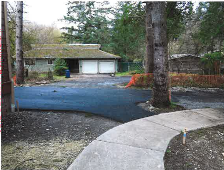
Asphalt abutting sidewalk to homes and extending into the turnaround that is on WLCH property
