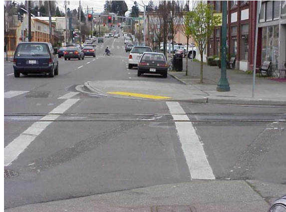
Bulbout at 4 th and Jefferson reduced crossing from 3 lanes to 2.
