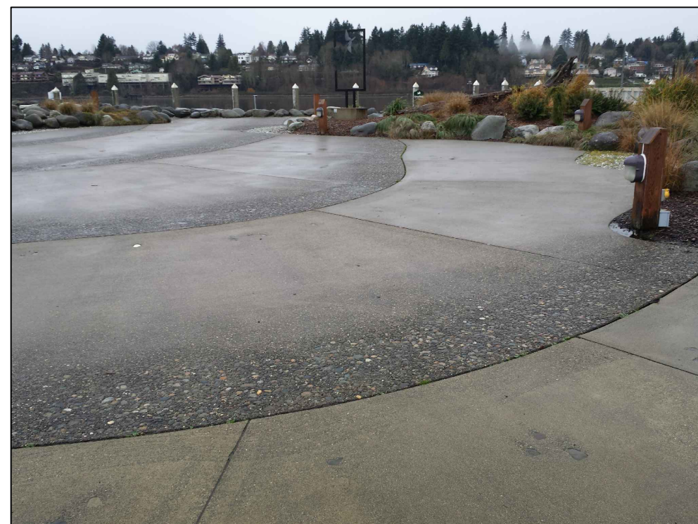
Beach-look exposed aggregate concrete
