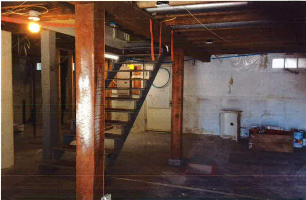
3 Ground level at West entrance 2015
