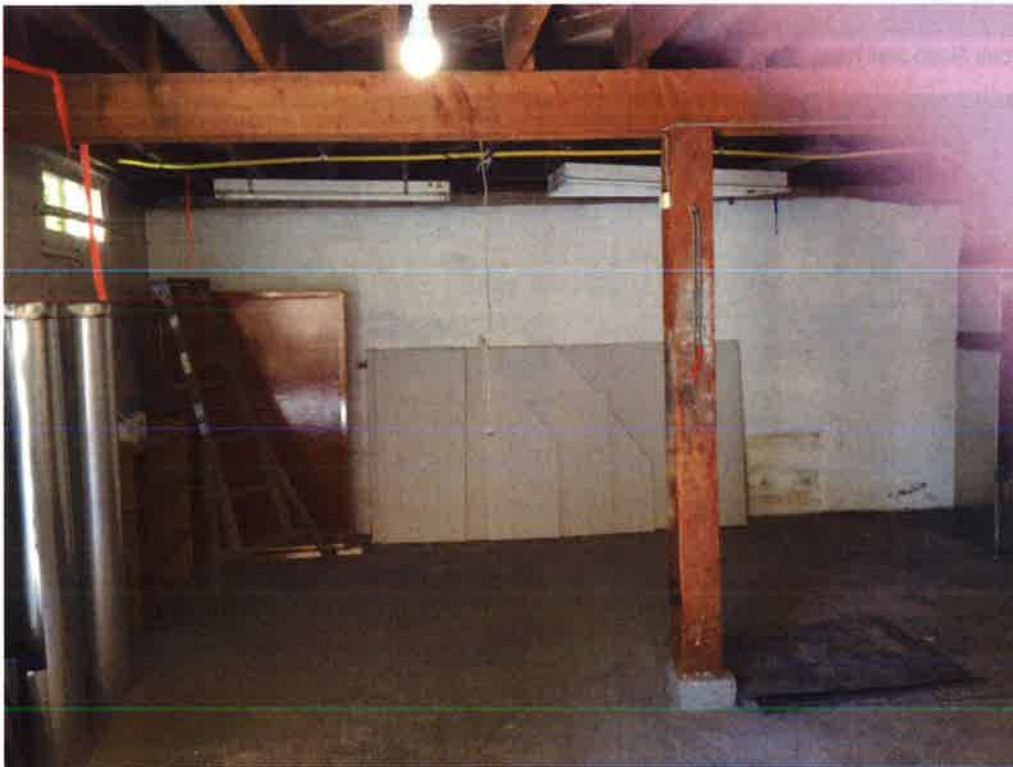
4 Ground level at West entrance looking left 2015
