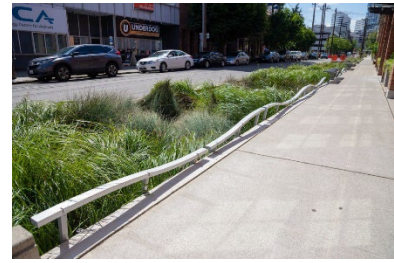
Figure 6-3. Main streets might include public-private stormwater partnerships like the Swale on Yale in downtown Seattle.
