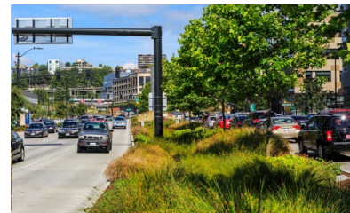
Figure 6-4. Bothell Way (Bothell, WA) and Mercer Street (Seattle). Arterials might include larger rights-of-way with additional greenery, larger stormwater facilities, and/or local collectors.
