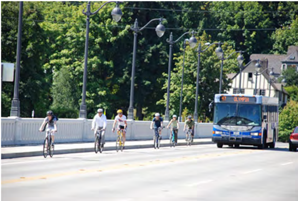
A bus travels over the 4 th Avenue Bridge.
