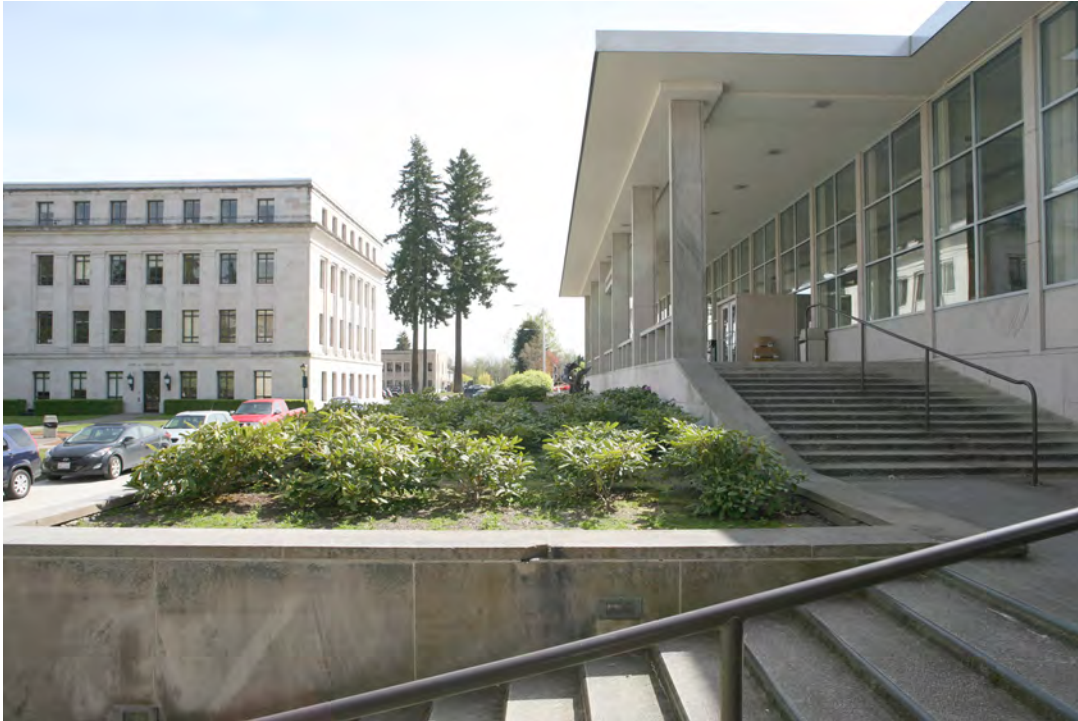
3 of 14. Washington State Library, front north facade looking east with the Cherberg Building in the background.
