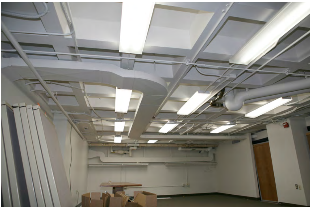
12 of 14. Washington State Library, typical waffle slab configuration in the rear stack volume.
