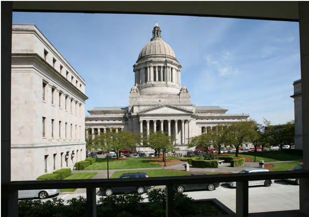
5 of 14. Landscape, view from the front of the Washington State Library looking north towards the Legislative Building.
