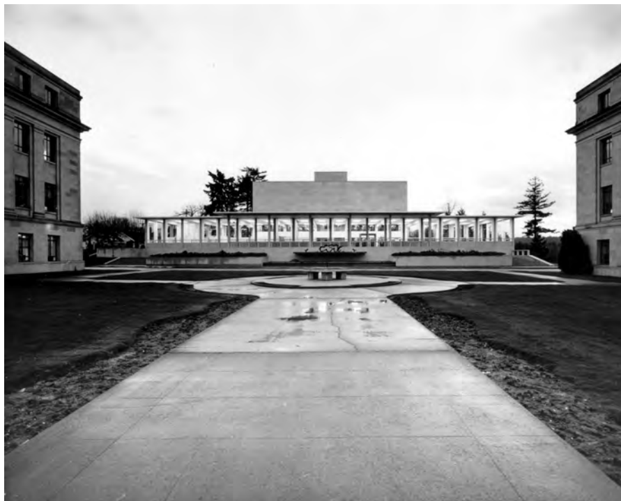
11. Ca 1959 view of the Washington State Library and the sundial plaza framed between the Cherberg and O'Brien buildings. Source: Washington State Library
