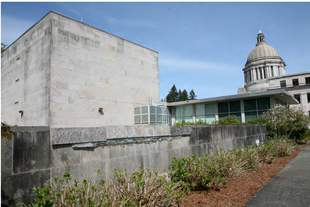
2 of 14. Washington State Library, southeast facade showing the rear stacks.
