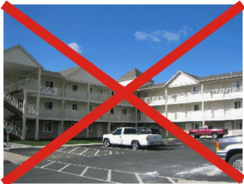
Figure 18.120.230.B.2. Elevated external walkways such as this are not allowed.
