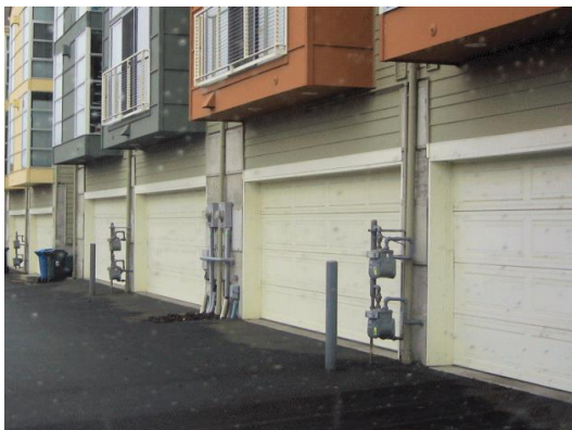
Figure 18.120.260.B.2: Place utility meters in less visible locations. Note that this example is acceptable on a service alley but not near a street or residential walkway.
