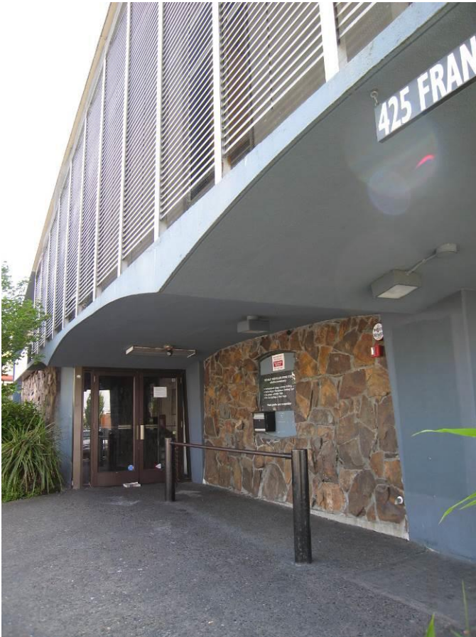
West façade showing secondary (parking lot entrance).
