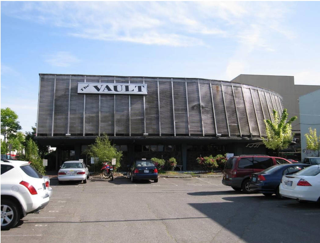
North façade showing rear sunscreen and curved rear façade. Drive through teller area is to the right.
