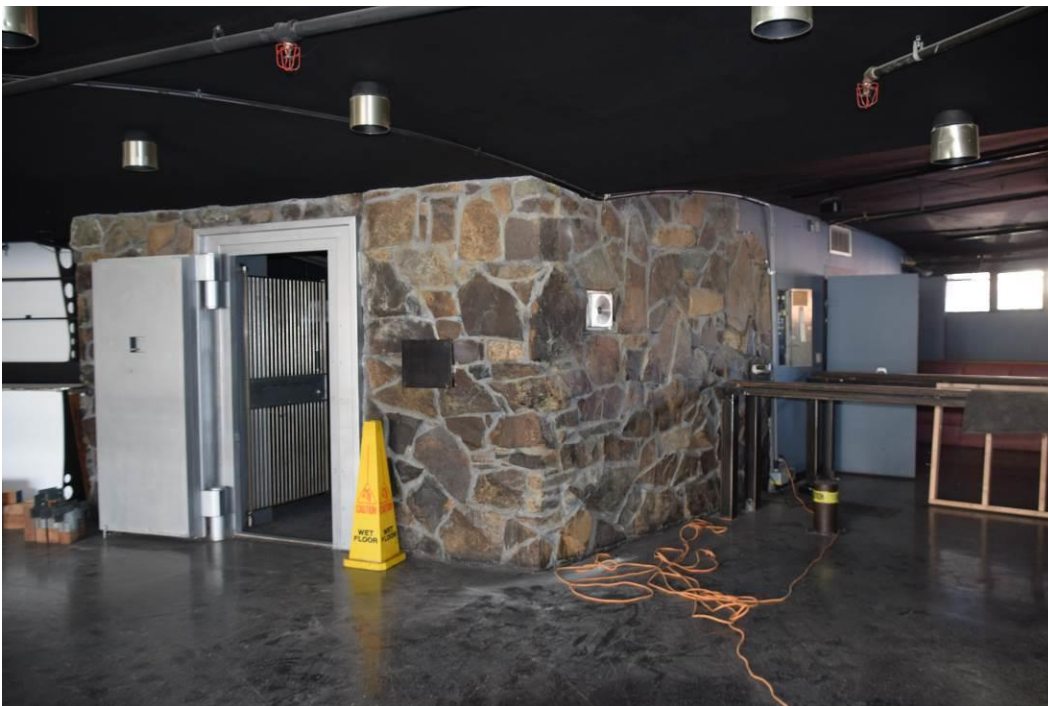
Detail of main banking vault.
