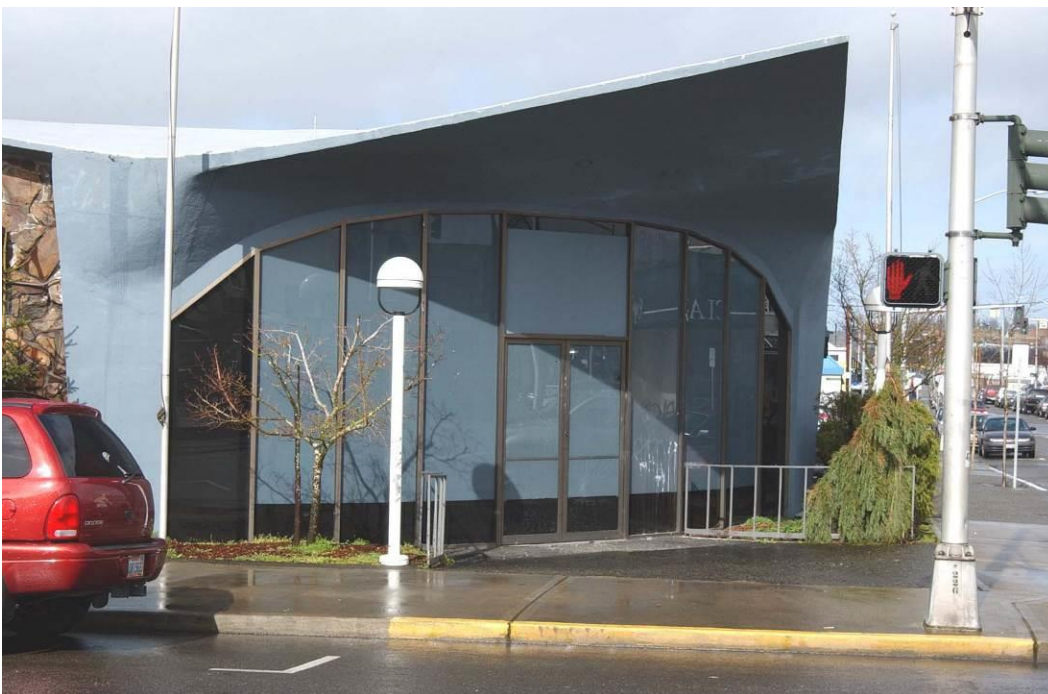
Detail of main bank lobby entry portal.
