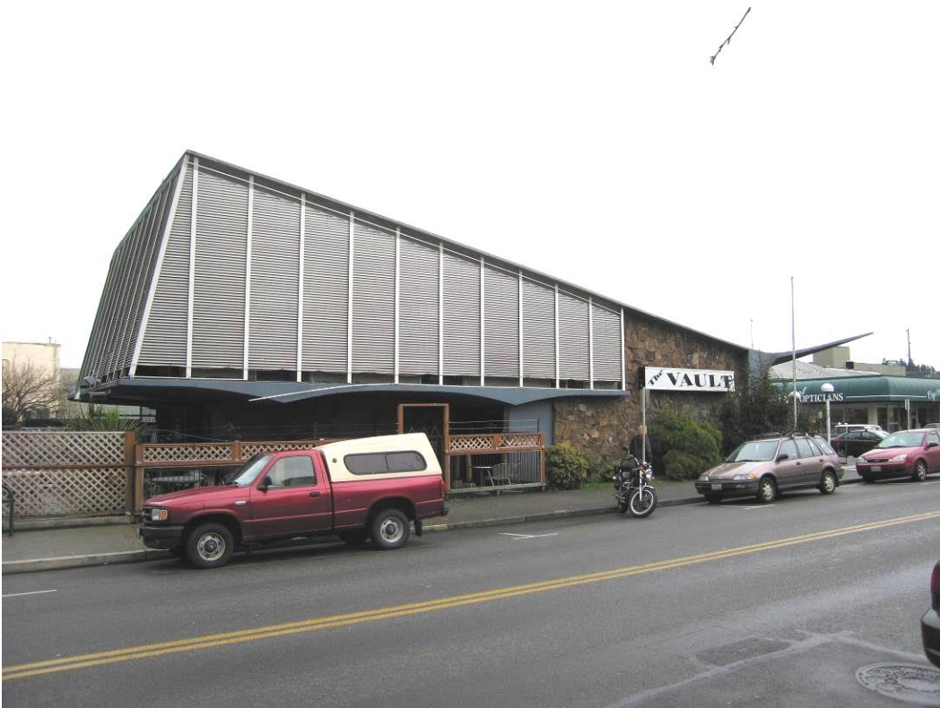
South façade showing rear sunscreen and barrel vaulted second floor decking system.
