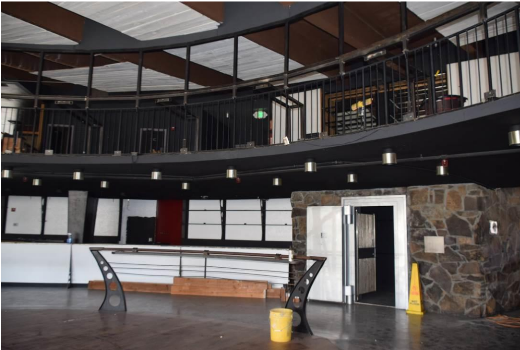
Banking lobby. View towards second story mezzanine area.
