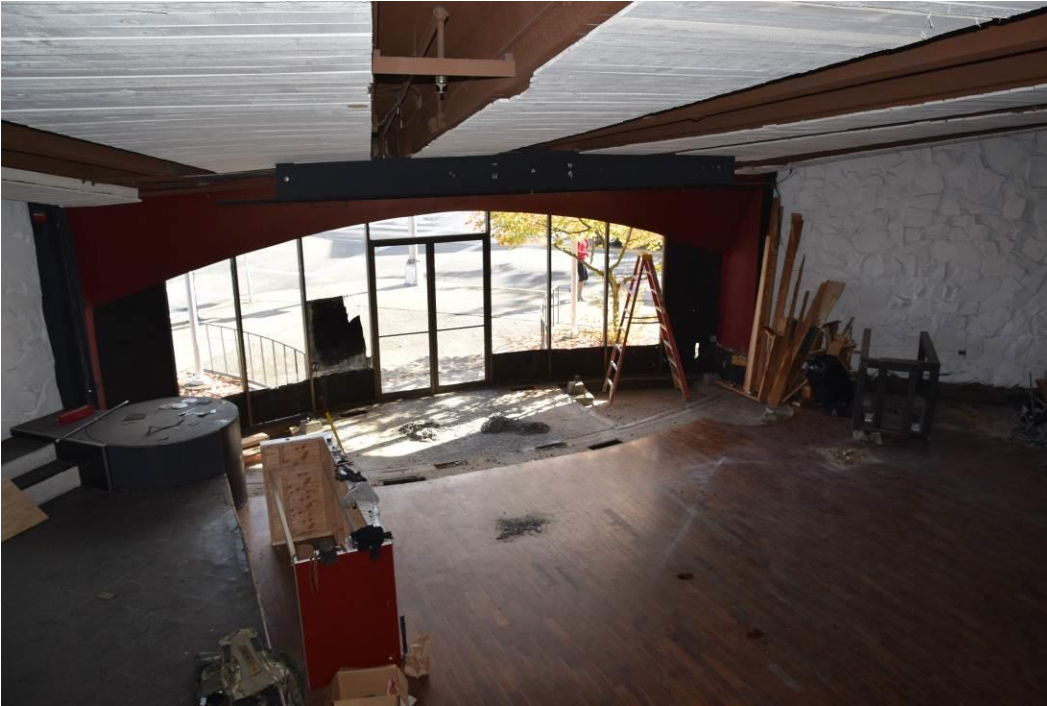
Banking lobby. View from second story mezzanine area towards main entrance.
